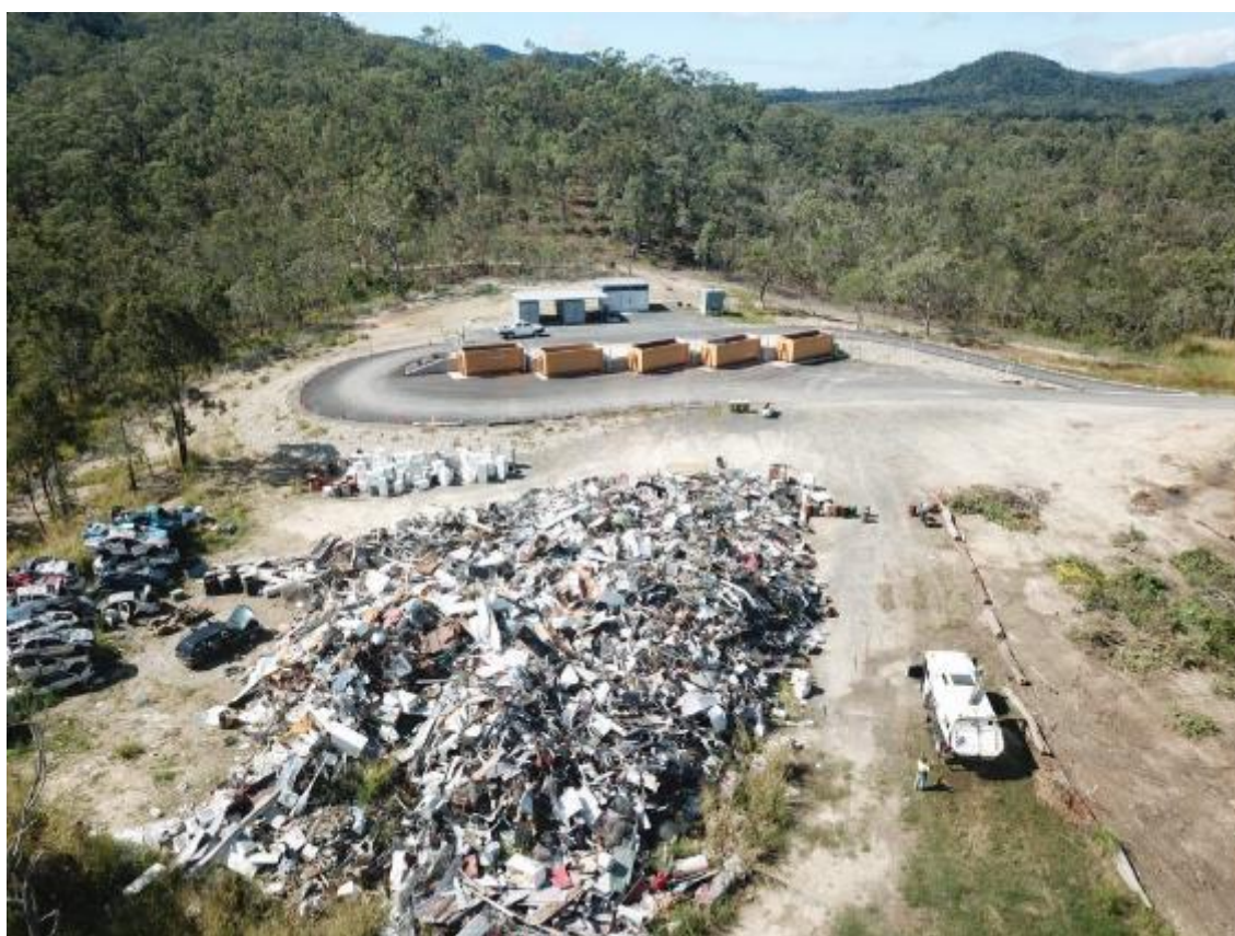
Figure 15 Upgraded Kuranda Waste Transfer Station 2017
