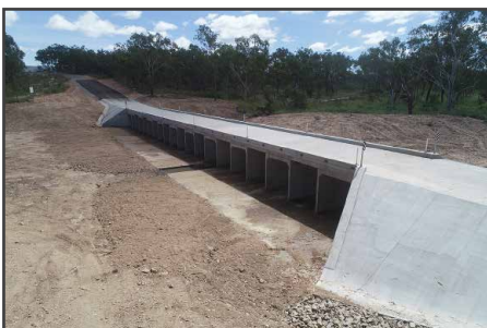
The James Creek Crossing on Wolfram Road, Dimbulah was replaced in April 2019. The crossing suffered significant damage from flooding in March 2018 and as a result Council applied for disaster assistance to replace the infrastructure.
