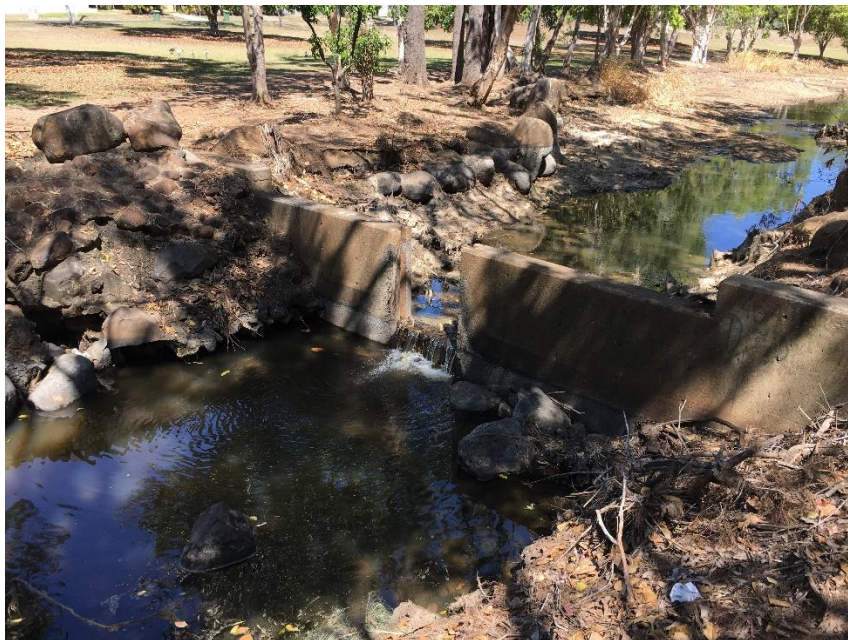
Weir with slats removed
