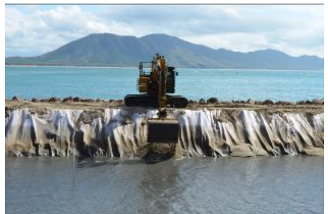
Eco-friendly solution – geofabric will minimise sediment loss from new seawall.
