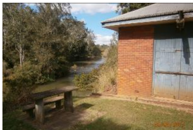
The Atherton Pump House on the Barron River.
