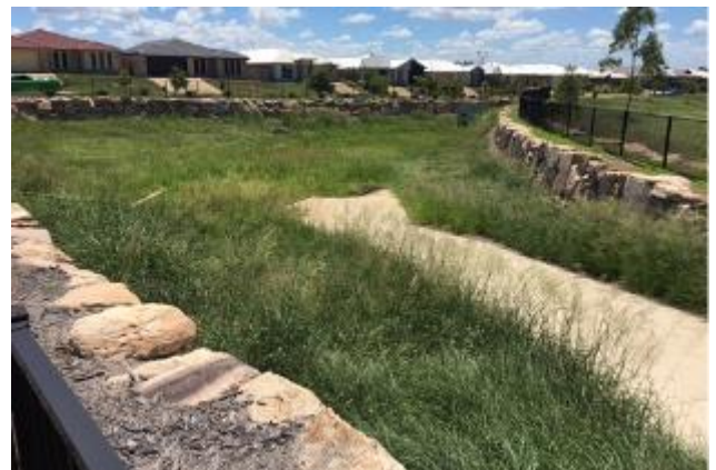
Putting Water Sensitive Urban Design into practice; a bio-swale in Norman Gardens, Rockhampton.
