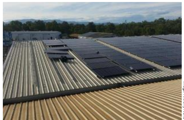
Solar panels power council depot.
