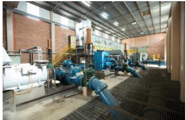
Upgraded facilities have major impact on energy efficiency.
