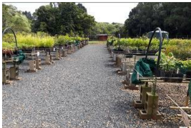
Improved surface drainage at revegetation nursery.
