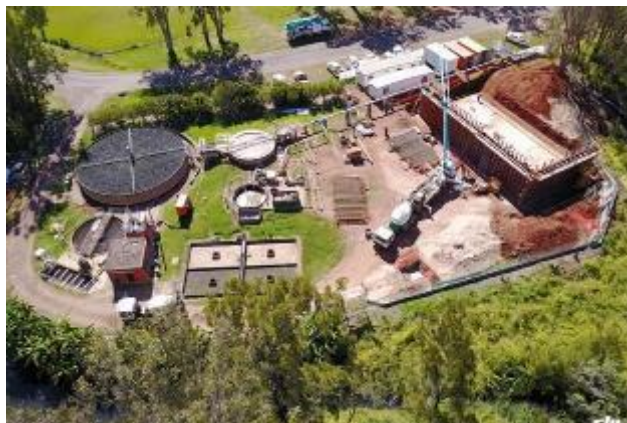
Bird's eye view of upgrades to the Ravenshoe Waste Treatment Plant, near the Millstream River.
