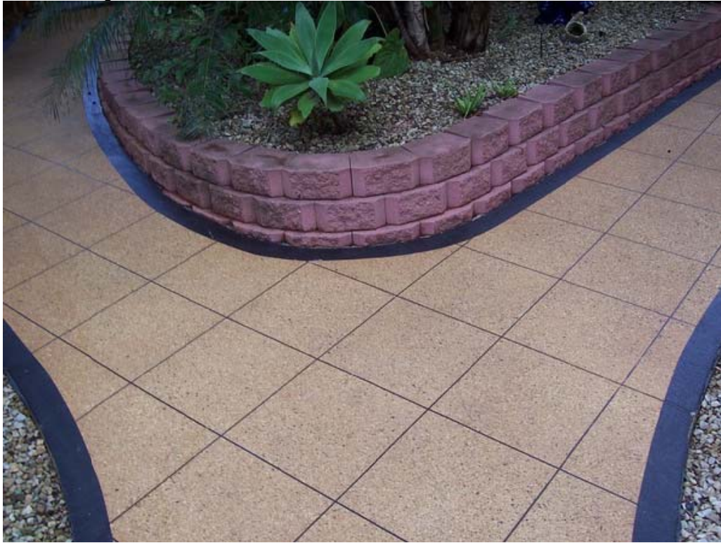
Mareeba - Figure 5.1.1 - Patterned Concrete
