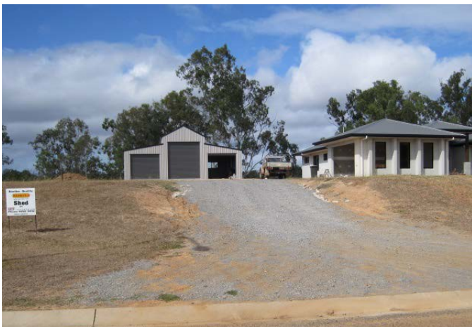
Figure 2 - A rumble pad constructed of large gravel to the entry /exit of the building
