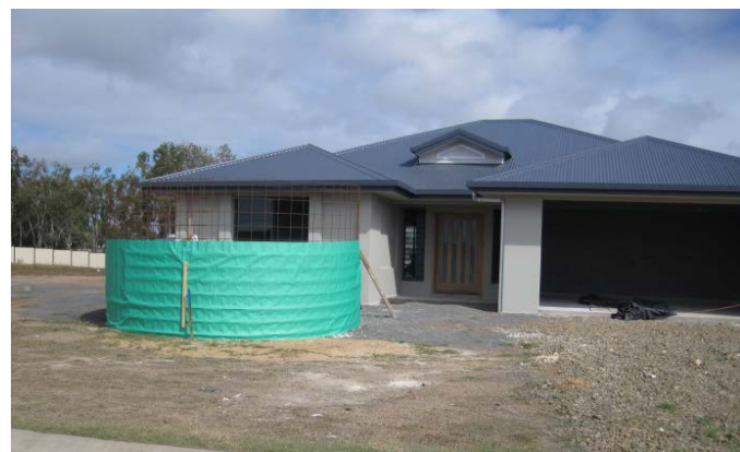
Figure 1 - A waste enclosure with a shade cloth surround to stop all waste being blown off site
