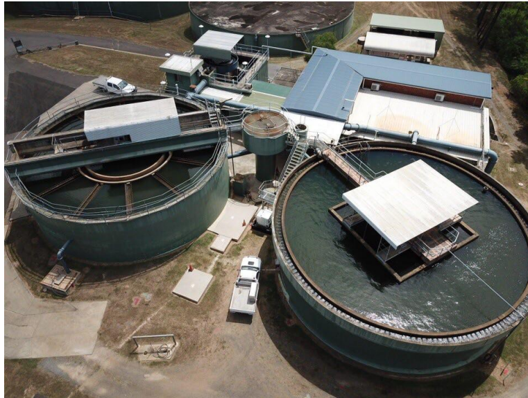
FIGURE 5: MAREEBA WATER TREATMENT PLANT
