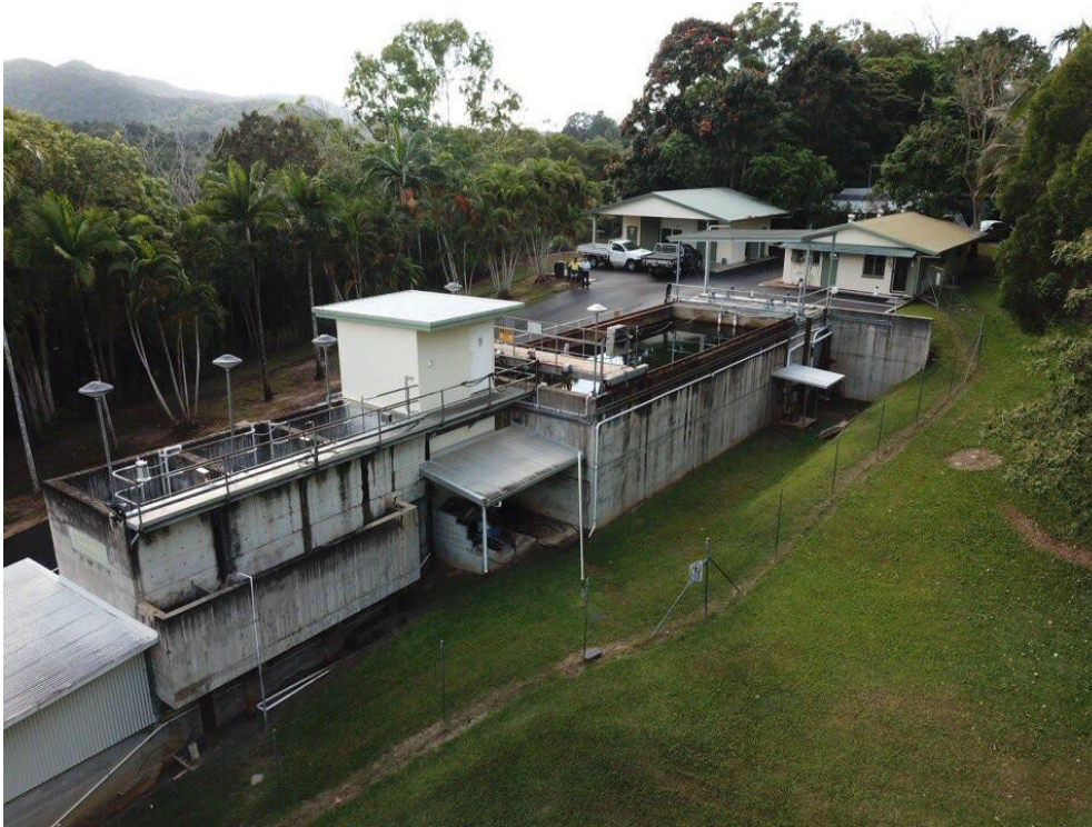
FIGURE 6: KURANDA WATER TREATMENT PLANT
