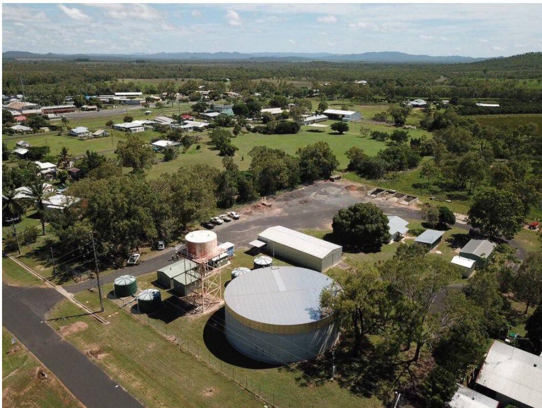
FIGURE 4: DIMBULAH WATER TREATMENT PLANT
