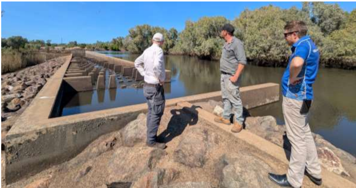
High-performance fish ladder at Glenore Weir
