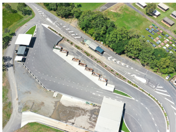
Mareeba Transfer Station Redevelopment, 2021
