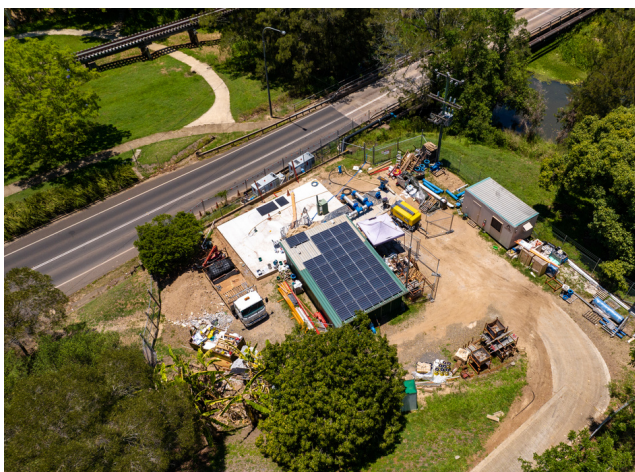
Granite Creek Pump Station upgrade, 2022
