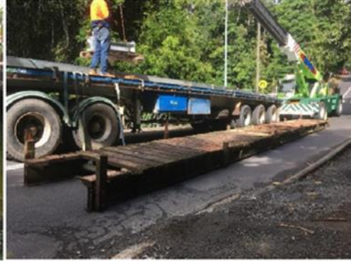
Old Barang St Pedestrian Bridge - Removed
