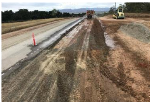
Installation of base gravel in widening
