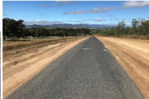
Completed subgrade between McBean & Stanton Roads
