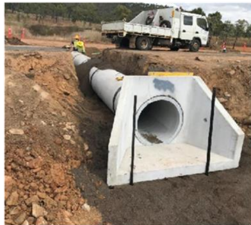
Newly installed culvert
