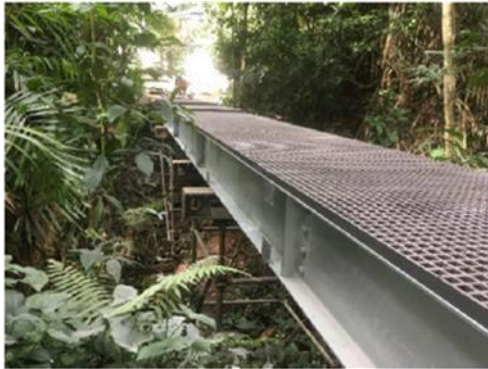
New Barang St Bridge - Under Construction
