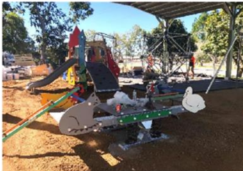
Installation of play equipment
