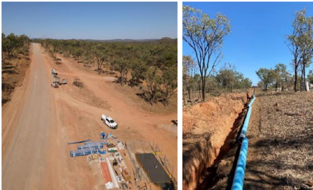
Bore shed, bore head works and pipeline construction
