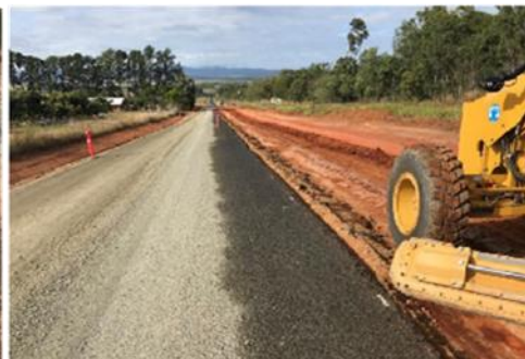
Clearing and the removal of existing shoulder material
