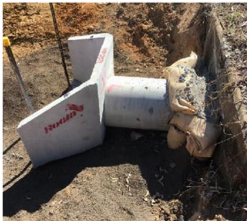
Existing culvert extension
