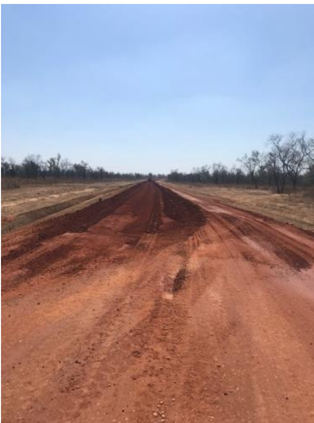
Mixing and Laying Process
