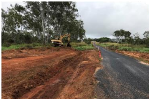
Drainage works at causeway site
