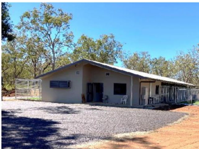
External Carpark seal complete
