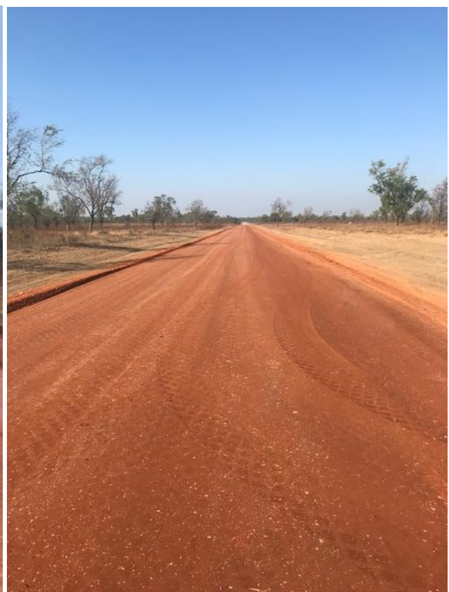
Completed Running Surface
