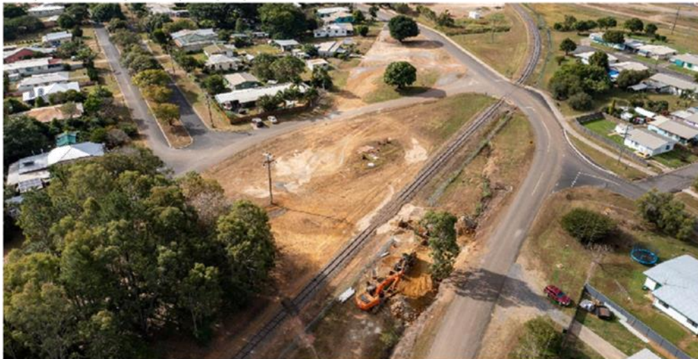
Installation of sewer main under Queensland Rail line near Perkins St
