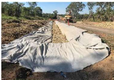
Replacing unsuitable material with rock and bitum
