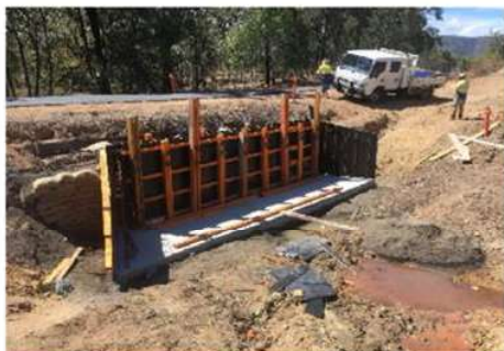
New headwall formwork
