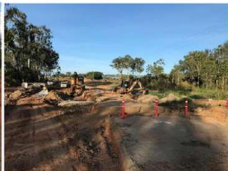
Preparation for culvert installation at Ch 3.60
