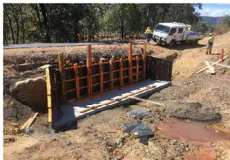
New headwall formwork
