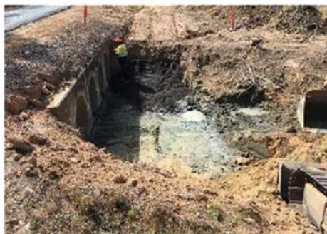
Preparation for major culvert extension
