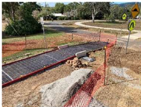
Culvert crossing adjacent to Fraser Road
