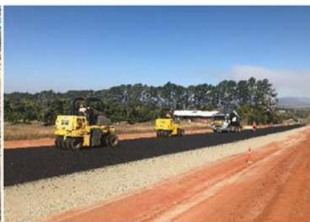
Sealing between McBean and Stanton Roads
