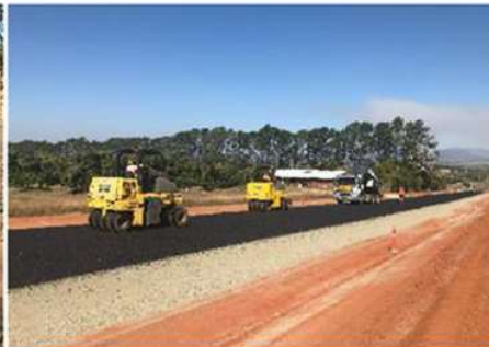
Sealing between McBean and Stanton Roads
