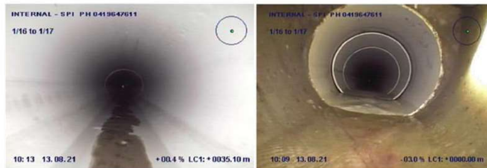
CCTV inspection footage on newly installed sewer main
