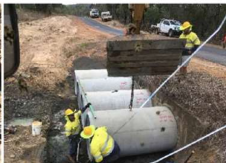
Installing RCP extensions
