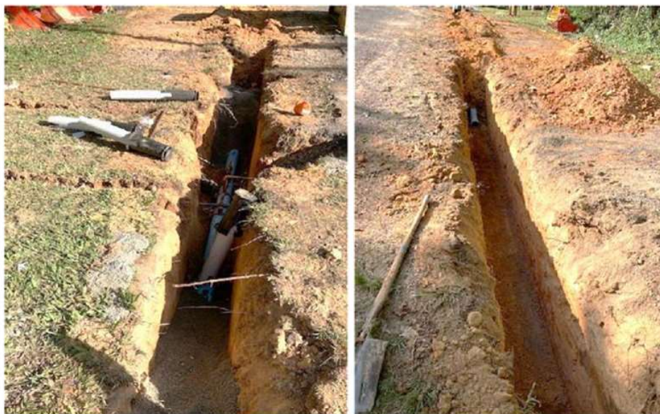
Newly pipeline construction and service connections
