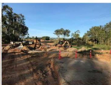
Preparation for culvert installation at Ch 3.60
