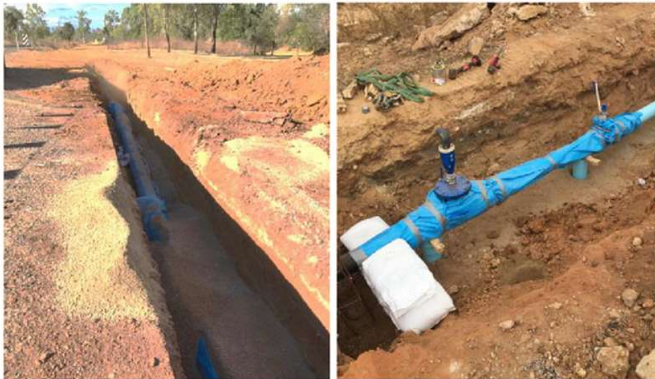
Newly road crossing pipeline in DICL construction and pipeline air release valve
