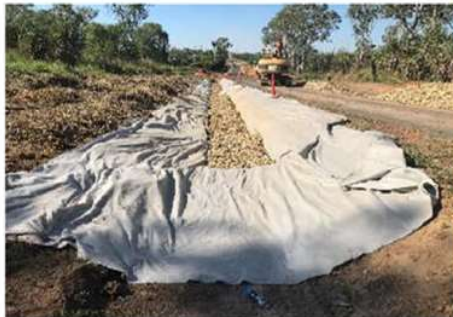
Replacing unsuitable material with rock and bidim
