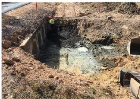
Preparation for major culvert extension
