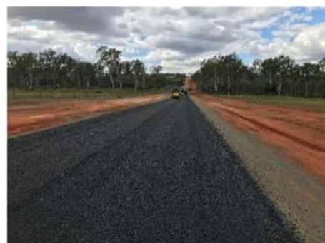
Sealing between McBean Road and causeway
