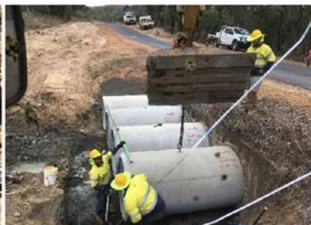
Installing RCP extensions
