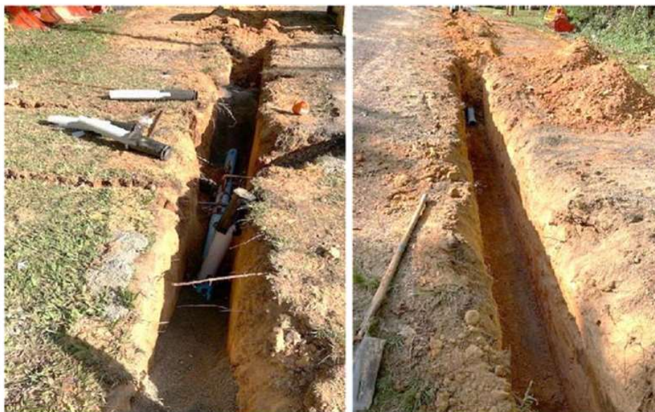
Newly pipeline construction and service connections
