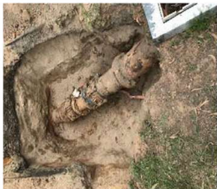
Existing flow meter prior to removal
