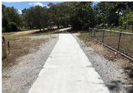
Upgraded concrete path at rear of houses on Fraser Road
