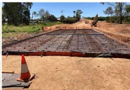
Widened causeway deck prior to pouring
