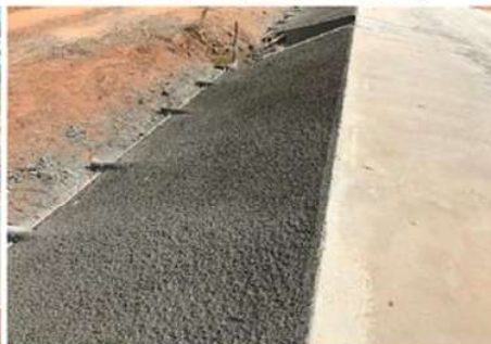
Causeway shotcrete batter protection
