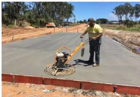
Causeway concrete finishing
