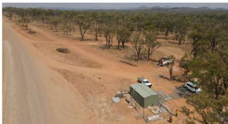
Newly constructed bore headworks shed
