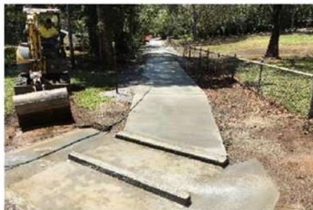
Culvert base and nib walls
