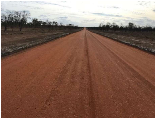
Completed running surface Ch 453
