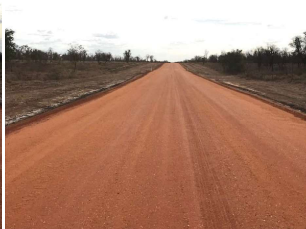
Completed running surface Ch 454
