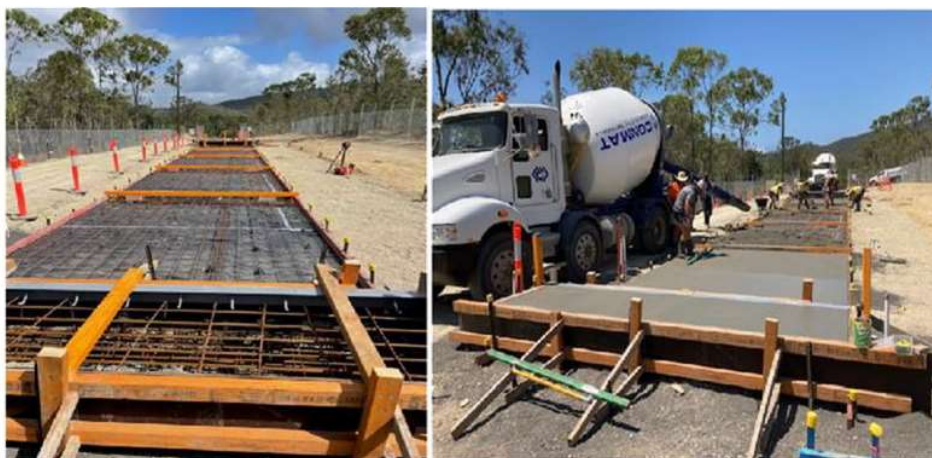
Weighbridge construction works
