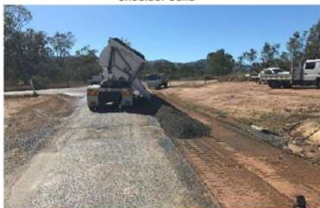
Filling with road base
