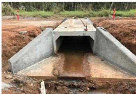
Widened causeway culvert wingwalls
