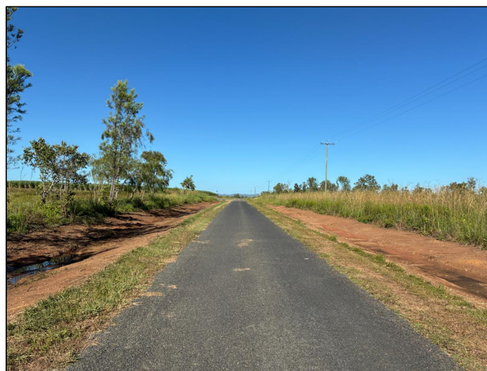
Stripping of table drains
