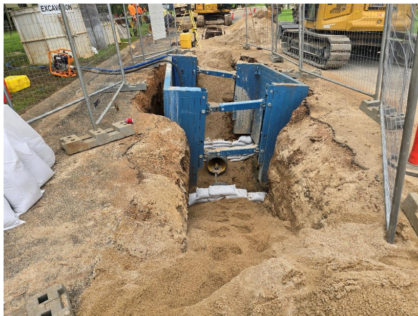
Trenching works continued along Constance Street
