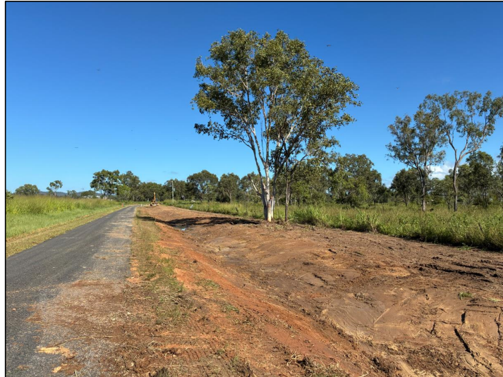
Stripping of table drains
