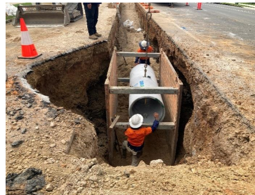
Constance Street Stormwater Pipe Trenching & Installation
