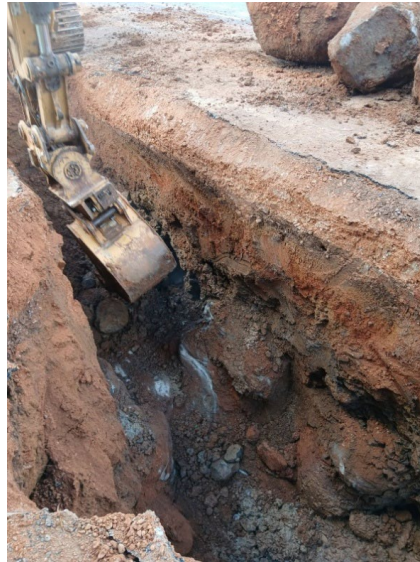
Trenching works continuing including through rocky conditions
