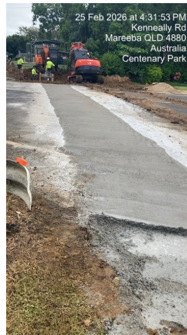
Completed works across Mareeba Connection Road
