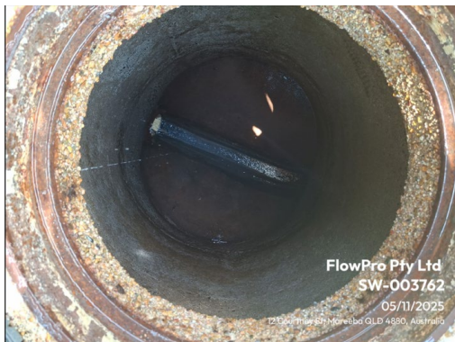
Before refurbishment works.
