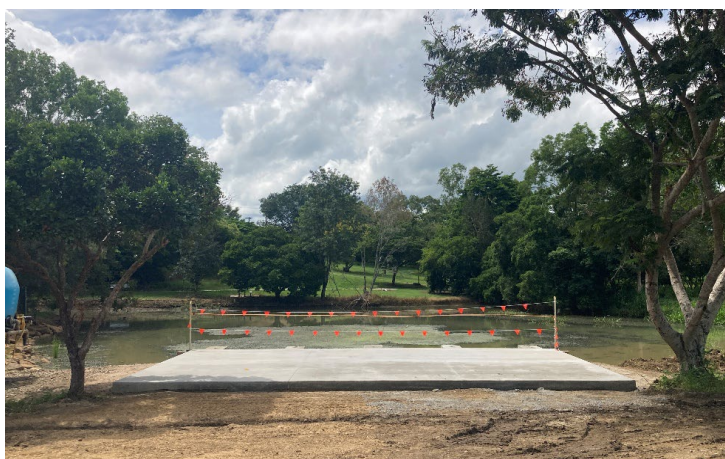
Concrete Deck Section Poured
