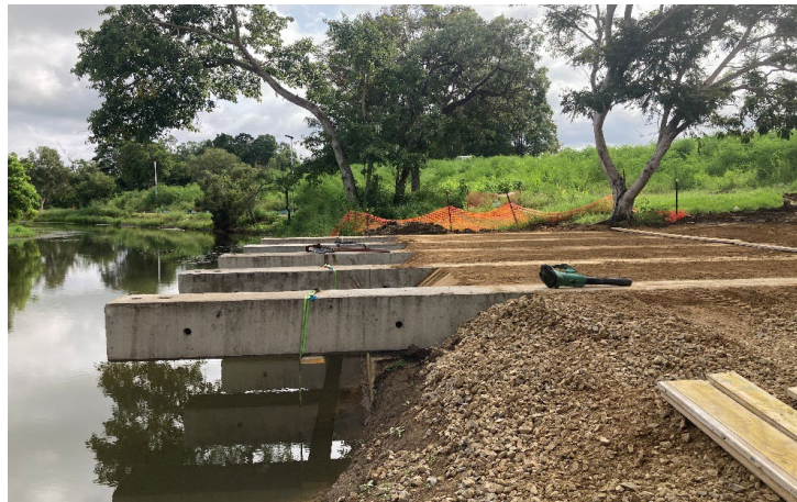
Cantilevered Deck Girders in Place
