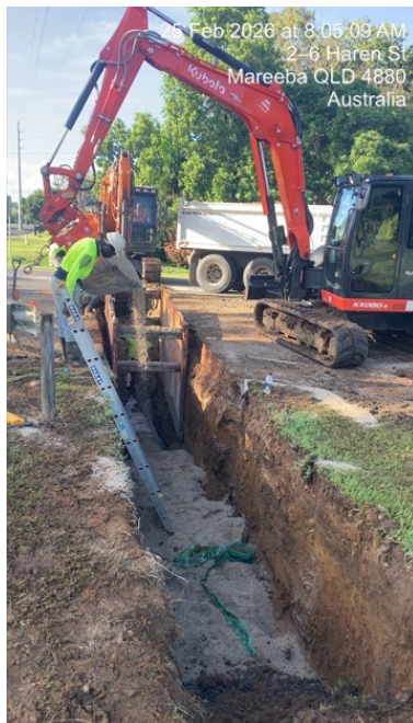
Works progressing across Mareeba Connection road
