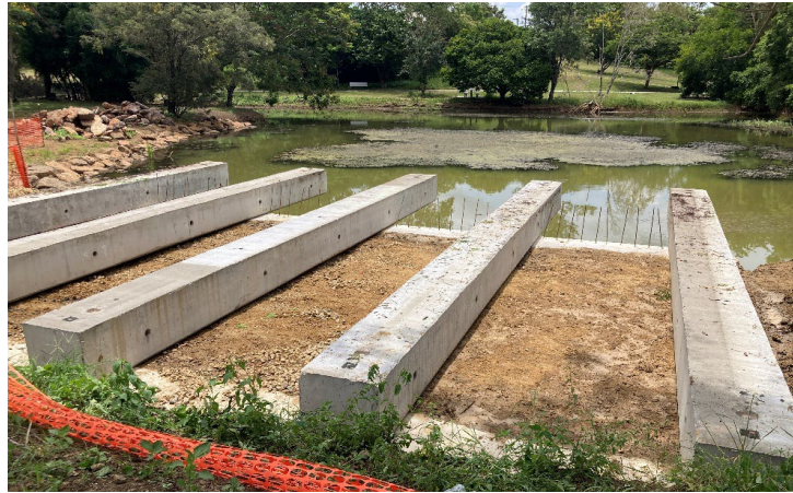
Deck Girders Craned into Place & Sitting on the Anchor Beams
