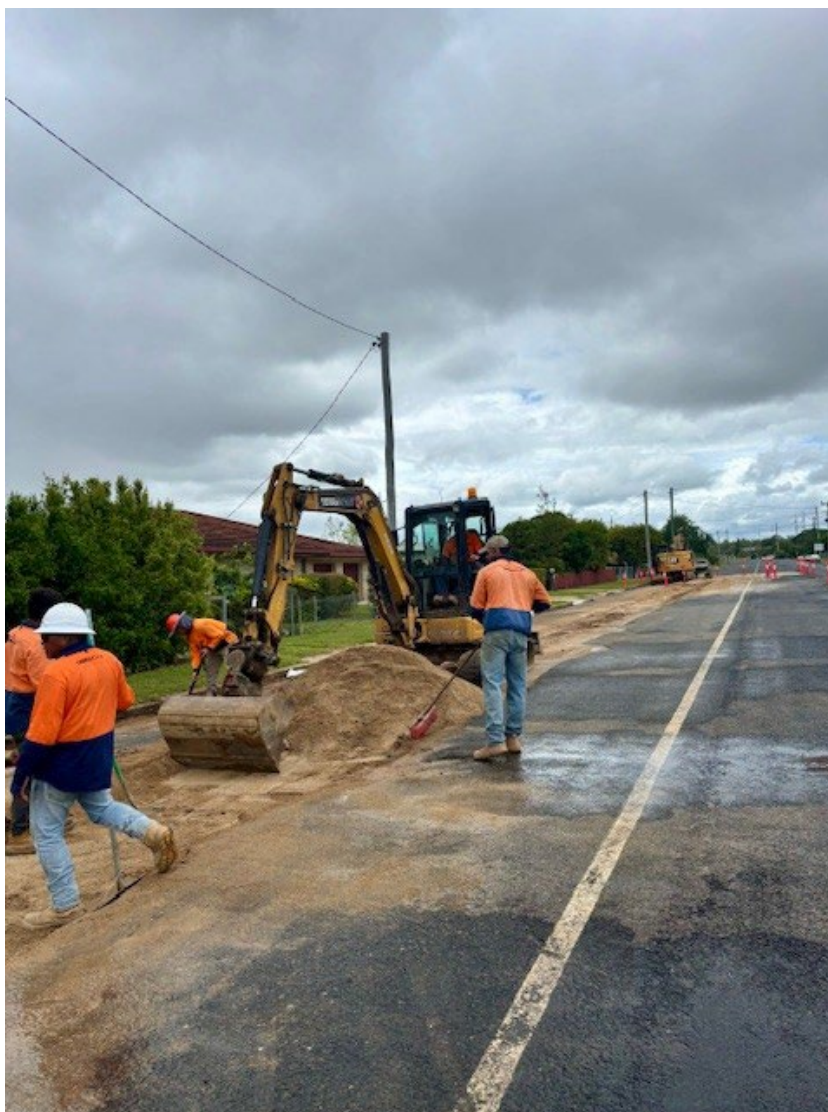
Sewer main installation works between Herberton Street and Basalt Street.
