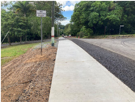
Bitumen Seal & Kerb Installation
