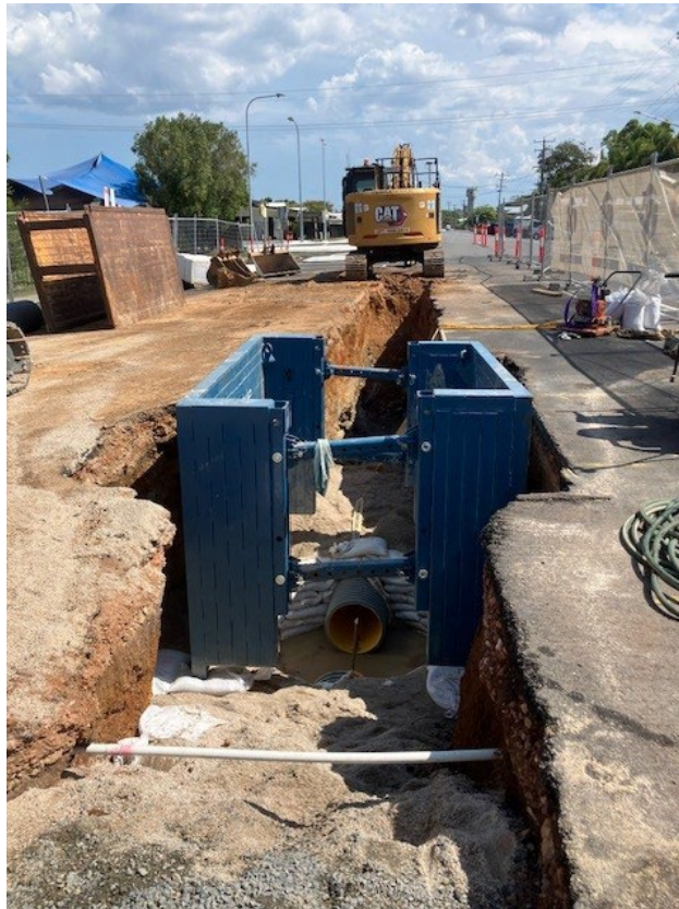
Constance Street Manhole and sewer pipe construction
