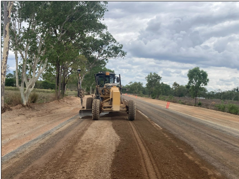
Laying and compacting gravel pavement
