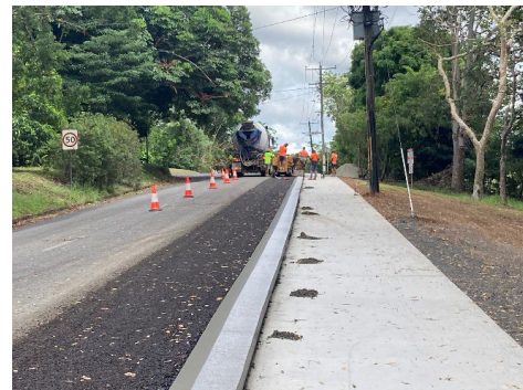
Bitumen Seal & Kerb Installation
