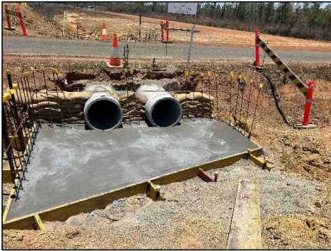
Apron and headwall works on pipe extensions
