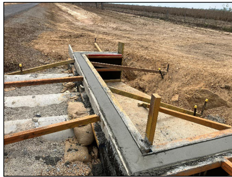
Apron and headwall works on pipe extensions
