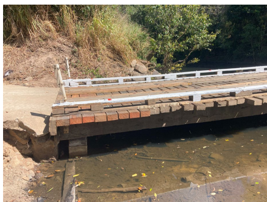
Raised abutment and decker replacement complete
