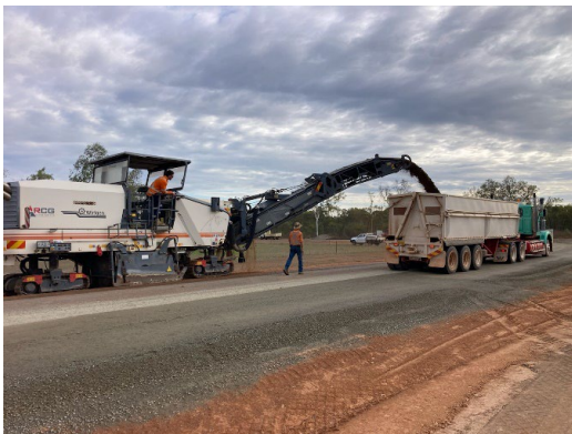
Milling out shoulder to depth
