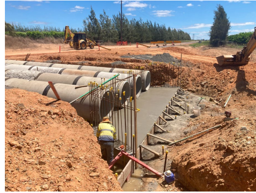
1200mm Diameter culvert, headwall and apron Installation
