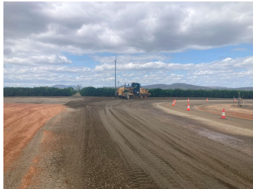
Laying and compacting base gravel
