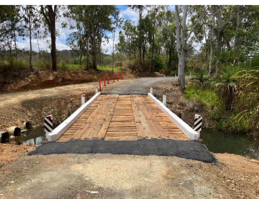
Timber bridge after repairs
