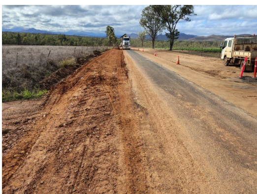
Extensions and shoulder reinstatement
