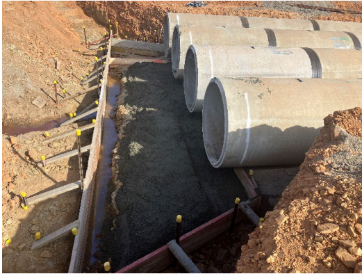
1200mm Diameter culvert, headwall and apron Installation
