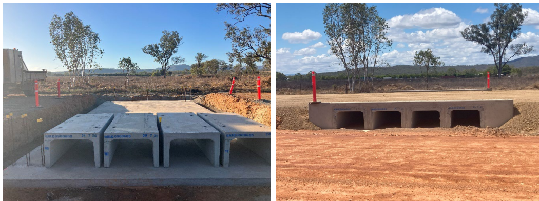
Installation of box culverts and backfill and cover with base gravel to road height
