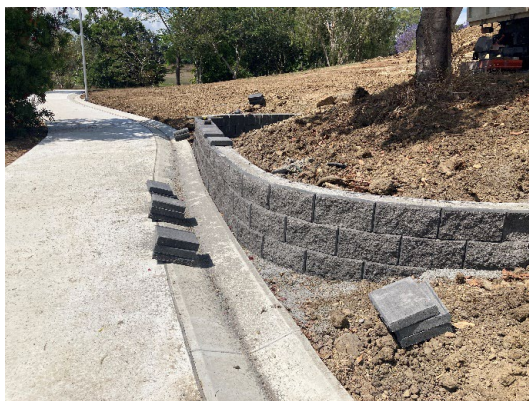
Retaining Wall Eastern Footpath
