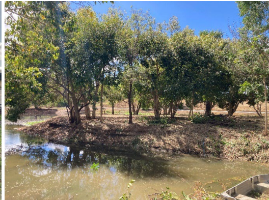
Clearing & Tree Trimming of the 'Central' Island
