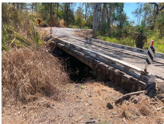
Timber bridge and girders before replacement
