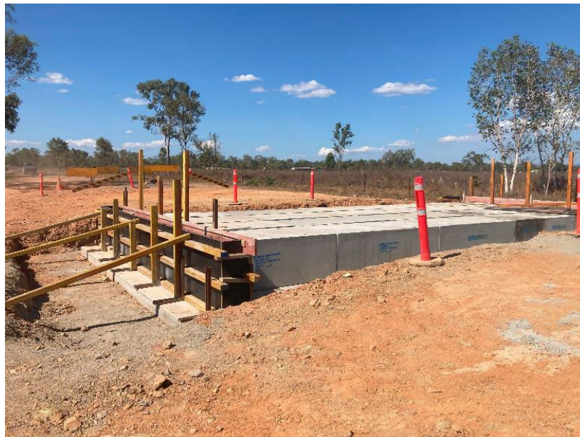
Installation of Box Culverts, and formwork for the headwalls.
