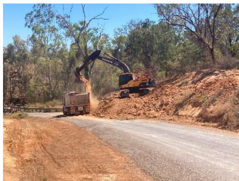
Batter removal Leadingham Creek Road, Dimbulah
