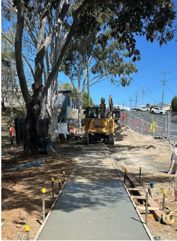
Works progressing along Constance St and footpath reinstatement.
