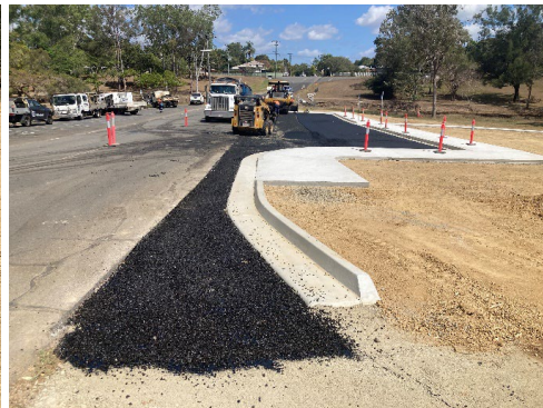
Carpark construction – gravel base material & asphalt surface
