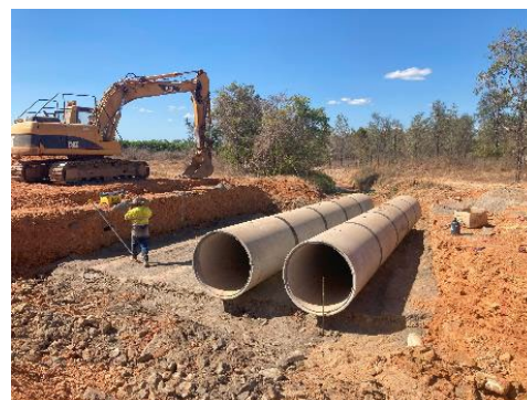
Installation of base material and 1200 diameter reinforced concrete culverts
