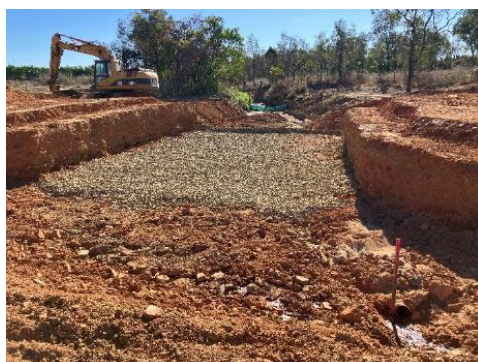
Installation of base material and 1200 diameter reinforced concrete culverts
