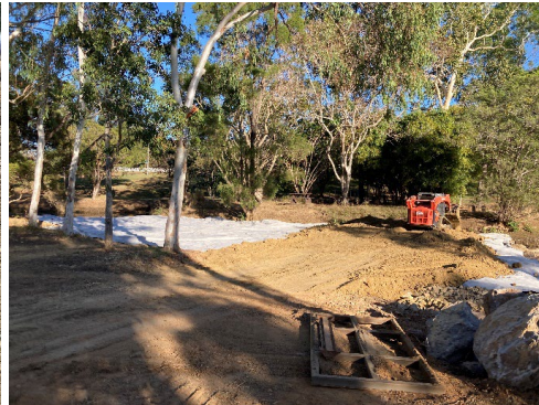
Reshaping and reclaiming stagnant section for a new footpath connection across the lake – larger rocks locked with 200mm shot rock & covered with geofabric and a clay layer
