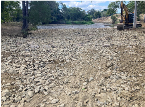
Reshaping and reclaiming stagnant section for a new footpath connection across the lake – larger rocks locked with 200mm shot rock & covered with geofabric and a clay layer
