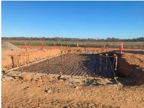
Reinforcing Mesh on Base Slab Leadingham creek Road, Dimbulah
