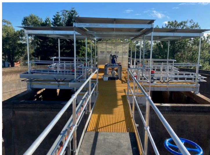
Installation of new walkway and chemical mixers.
