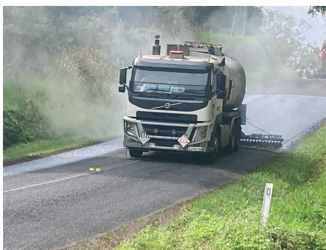
Bitumen Reseal, Speewah Road, Speewah
