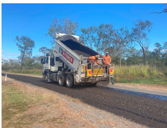
Bitumen Reseal, Volkman Road, Arriga
