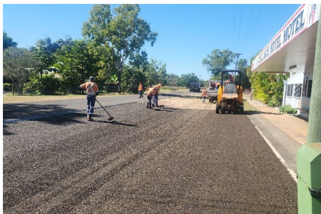
Bitumen Reseal, Tower St, Chillagoe
