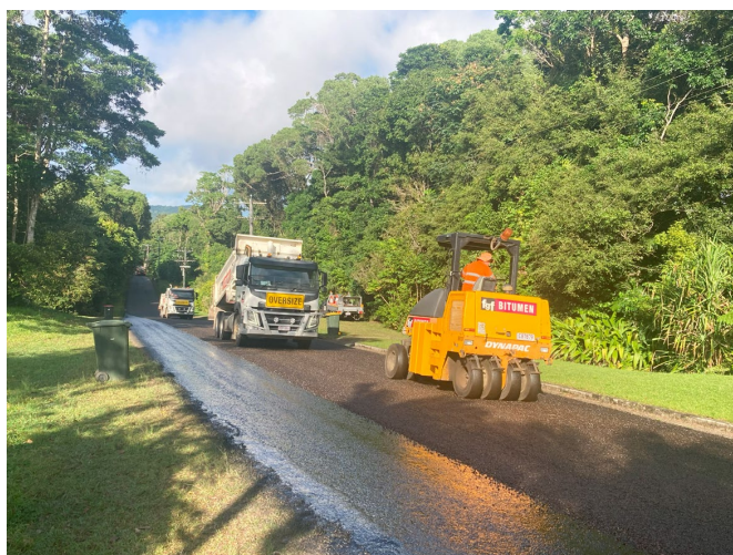
Bitumen Reseal – Barron Falls Road, Kuranda
