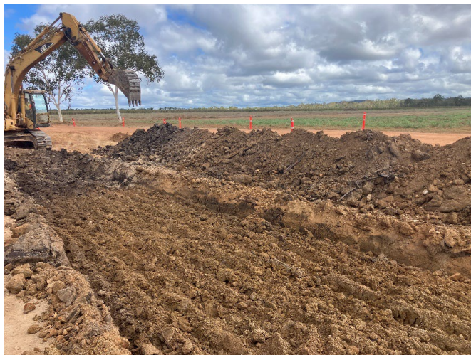
Removal of unsuitable material, Leadingham Creek Road, Dimbulah
