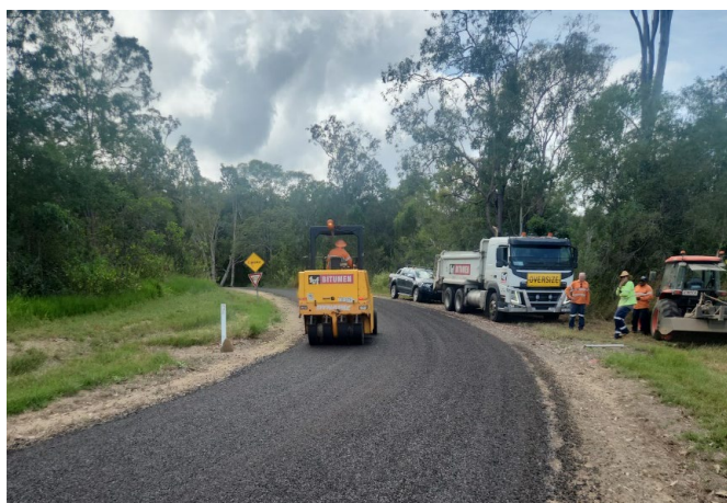
Bitumen Reseal, Bilwon Road, Bibbohra
