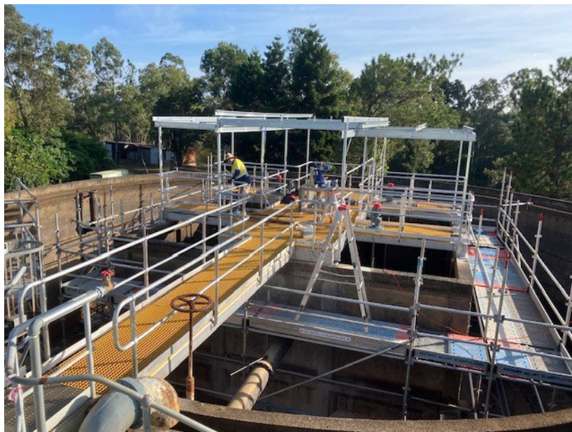
Installation of new walkway and chemical mixers.
