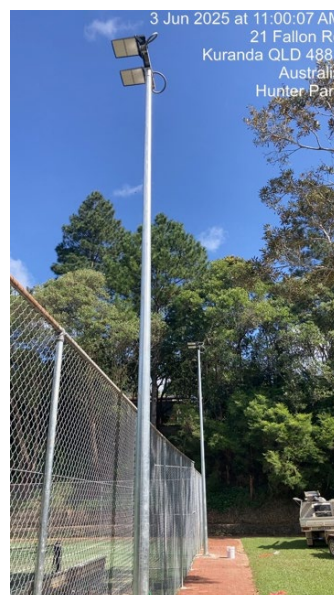
New lighting poles and LED lights installed to Australian Standards for Recreational use.
