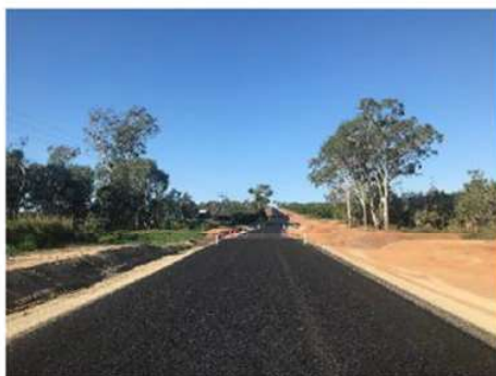
Completed Two Coat Seal
