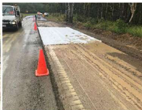
Geofabric put in place due to unsuitable subgrade
