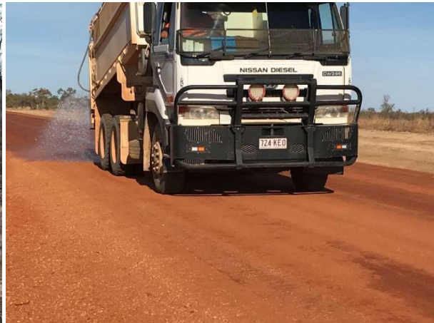
Back watering operation
