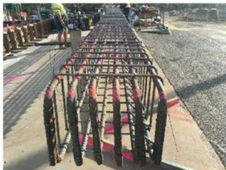
Girder Reinforcement
