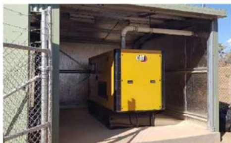
Newly constructed Motor Control Centre (MCC) for the Bore & Telemetry
