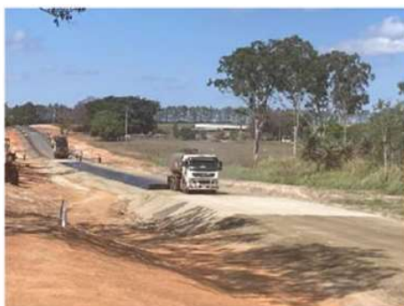
First Application of C320 Bitumen
