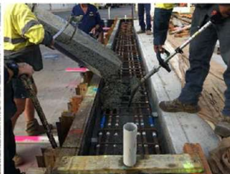
Pouring Concrete Girder
