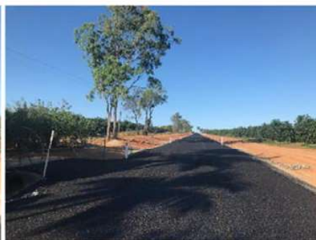
Completed Two Coat Seal
