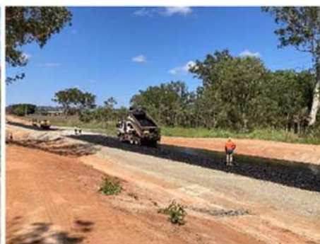
Spreading 16mm Aggregate
