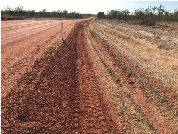
Completed running surface and table drain
