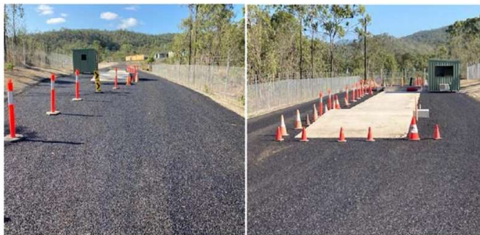
Weighbridge construction works
