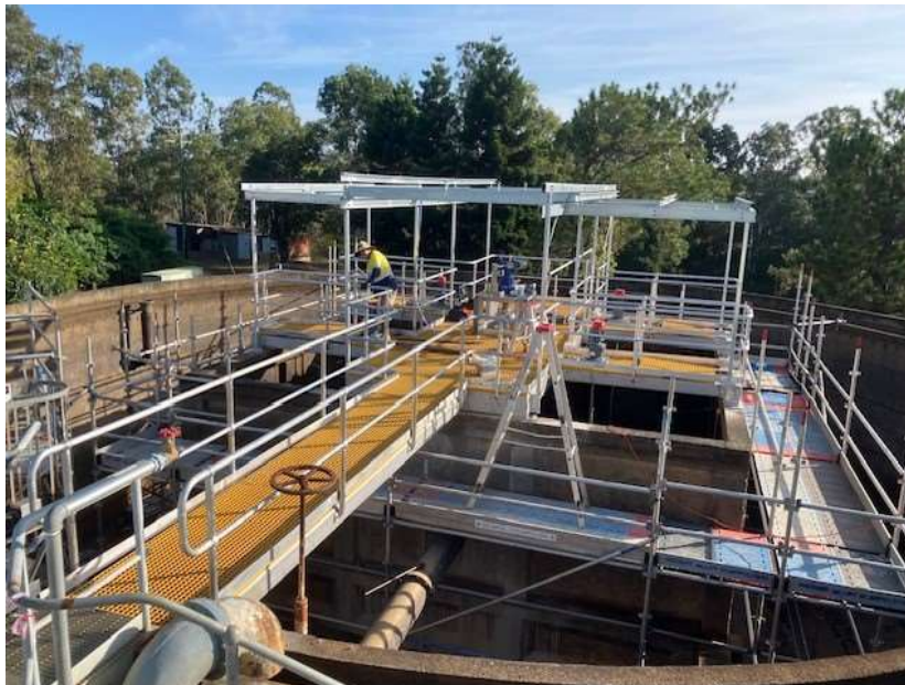
Installation of new walkway and chemical mixers.
