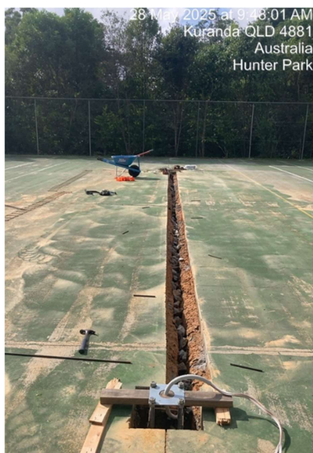
Trenching, cabling and footings for new light poles
