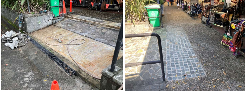
Dismantling, Reprofiting & Relaying a Section of Footpath & Ramp in Lower Coondoo Street
