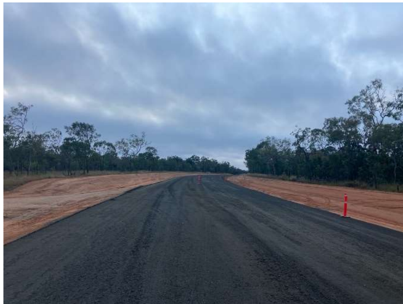
2.1 Road Base Gravel laid and compacted ready for final trim
