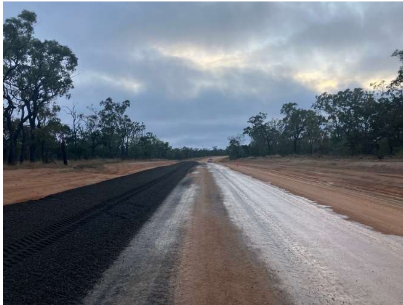
Moisture conditioned rill of 2.1 Road Base Gravel.
