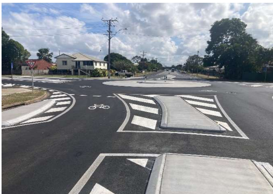
Line Marking and Road Furniture Installation
