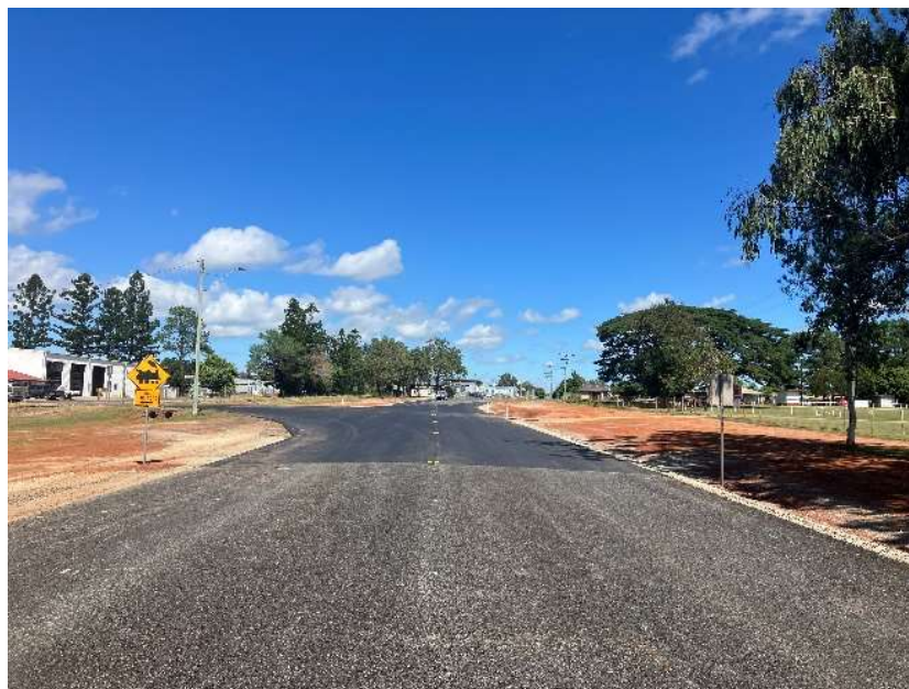
Asphalt Overlay Reynold St Intersection
