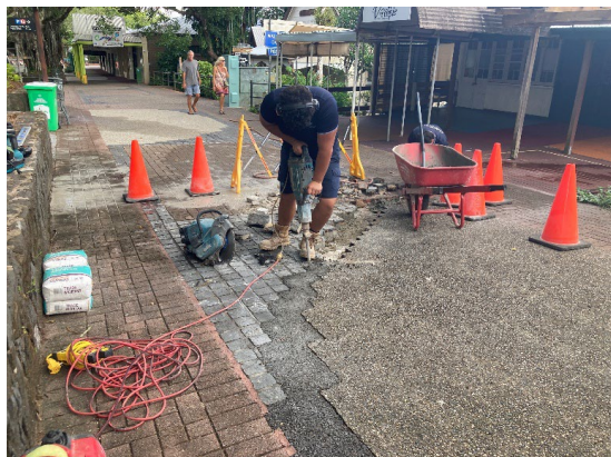
Replacement of Displaced Slab in Front of the Chemist - Corner of Coondoo & Thongon Streets
