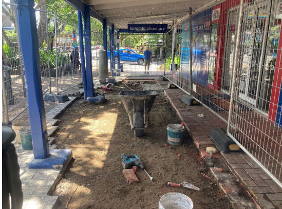
Replacement of Displaced Slab in Front of the Chemist - Corner of Coondoo & Thongon Streets
