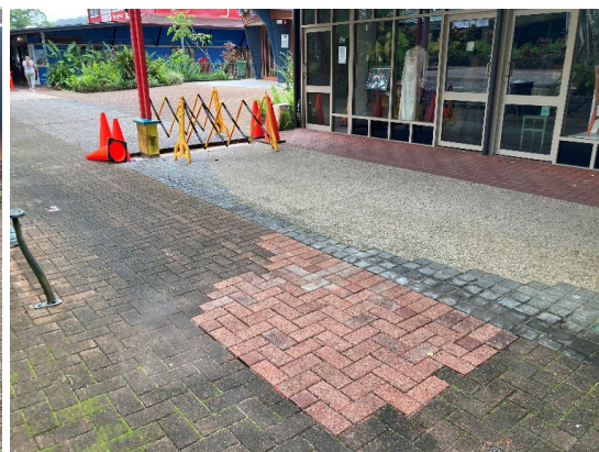
Replacement of Displaced Slab in Front of the Chemist - Corner of Coondoo & Thongon Streets
