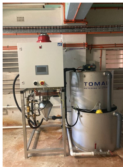
Installation of new chemical dosing equipment.
