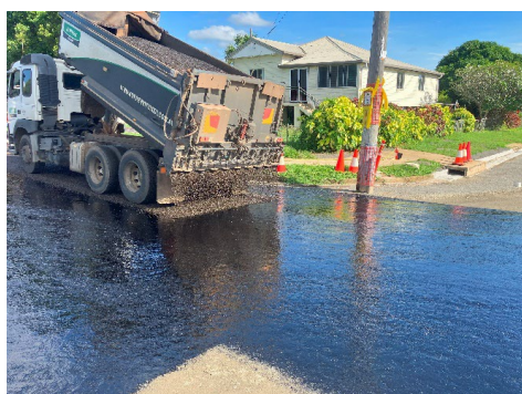
Bitumen seal
