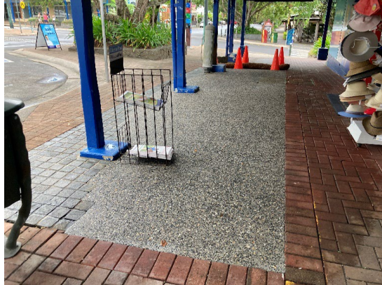
Replacement of Displaced Slab in Front of the Chemist - Corner of Coondoo & Thongon Streets
