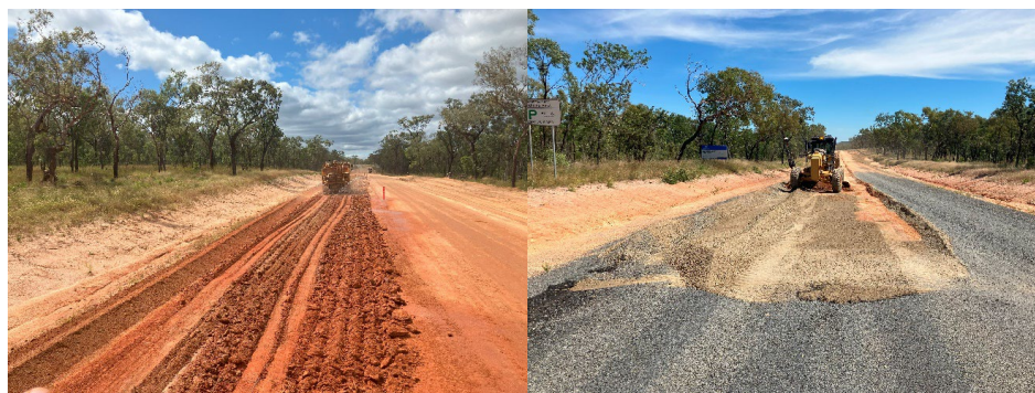
Watering existing subgrade prior to trimming
