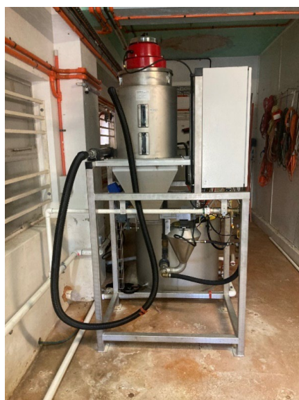
Installation of new chemical dosing equipment.
