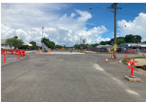
Base gravel – laid and compacted
