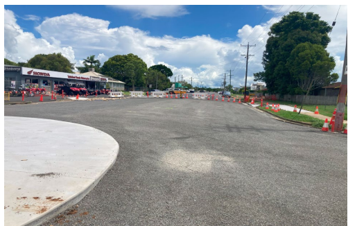
Base gravel – laid and compacted
