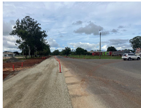
Base gravel in shoulder widenings
