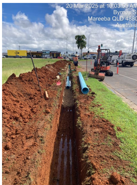
Installation of 225mm PVC Super Main. Byrnes St, Mareeba
