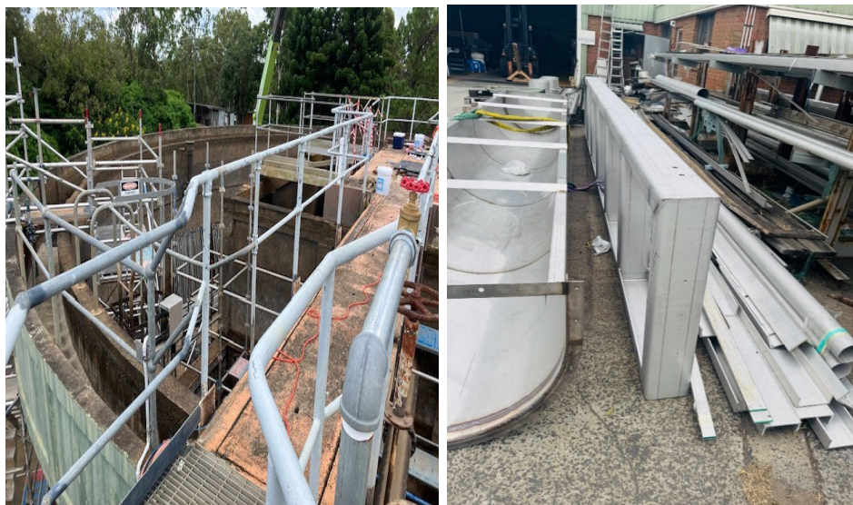
Stripping out Clarifier 1 and new equipment being manufactured.
