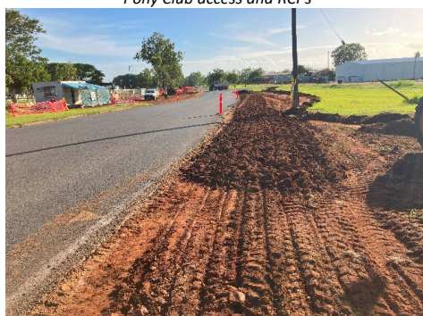
Drainage excavation – Reynolds Steet side
