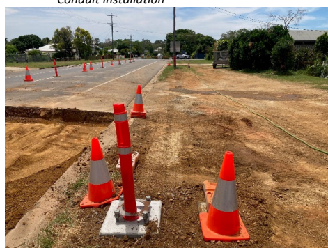
Completed rag bolt installation
