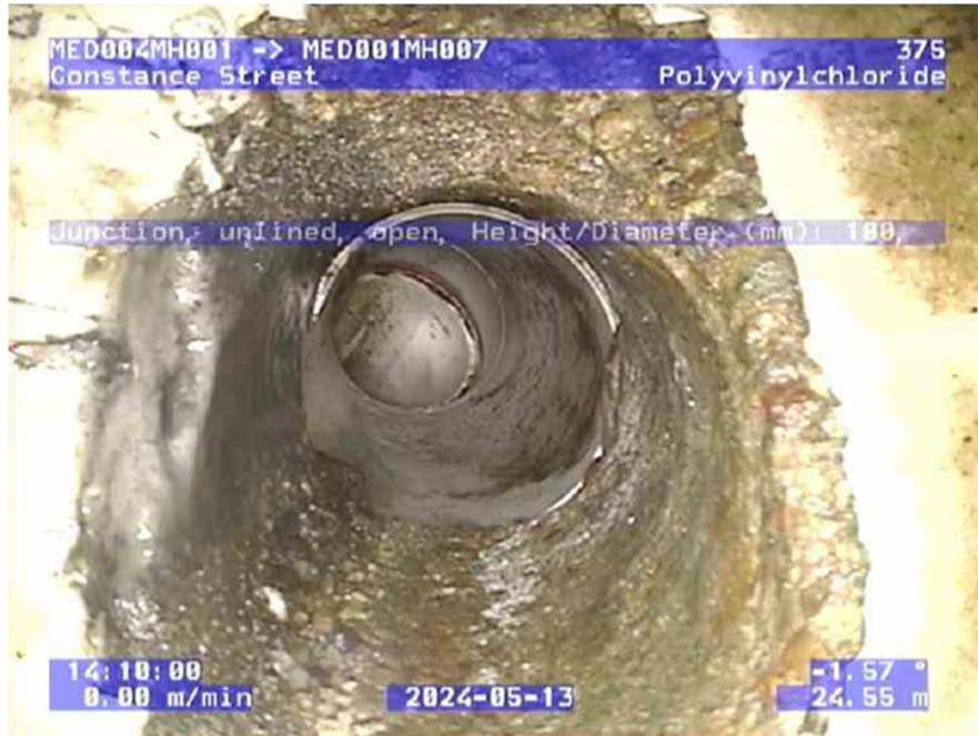
Captured image of identified defective sewer junction
