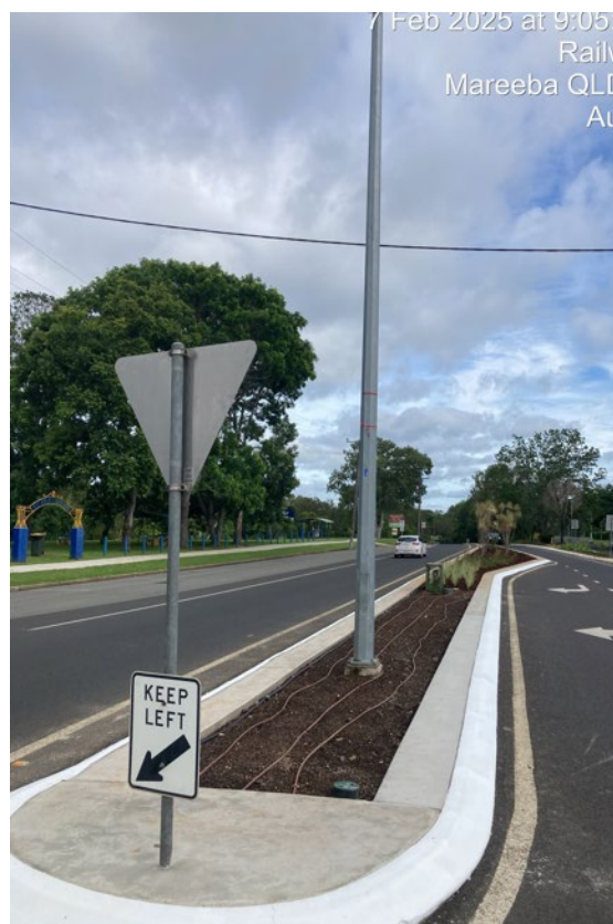
Location 7 – Granite Creek approach, Byrnes Street
