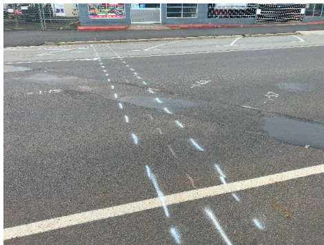
Marked trench for conduit
