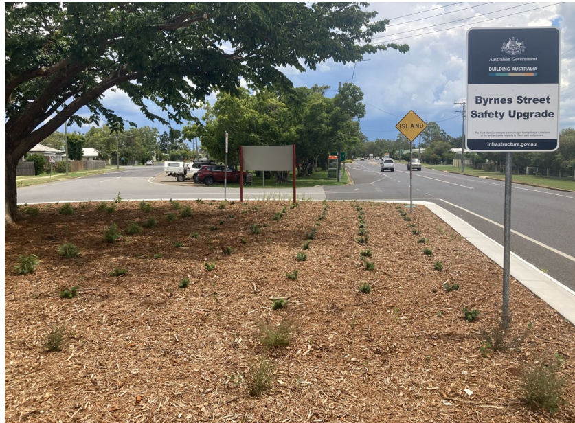
Location 2 - BP Median Island. Construction complete.
