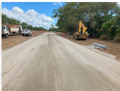
Completed base pavement layer
