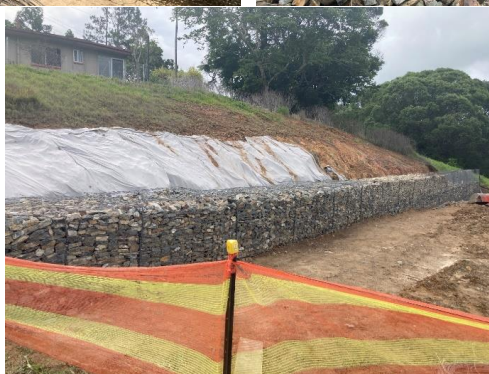
Gabion wall construction continuing
