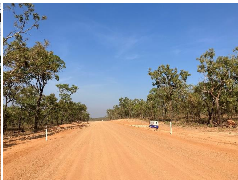
Ootann Road – after (subgrade level)
