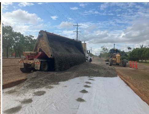
Tipping imported road base on bitum covered subgrade
