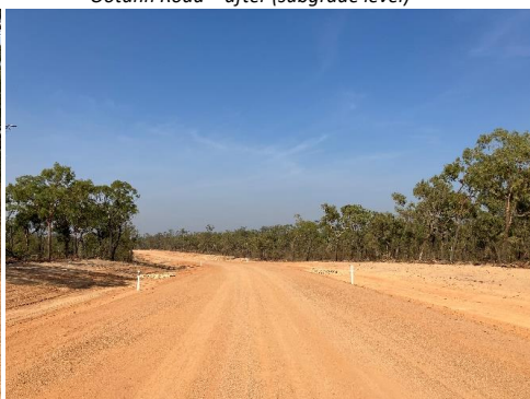
Ootann Road – after (subgrade level)
