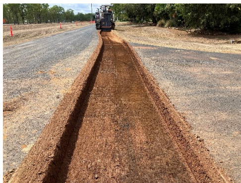
Removing existing failed pavement layer
