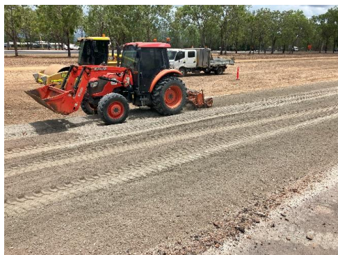
Blending bagged cement into base layer
