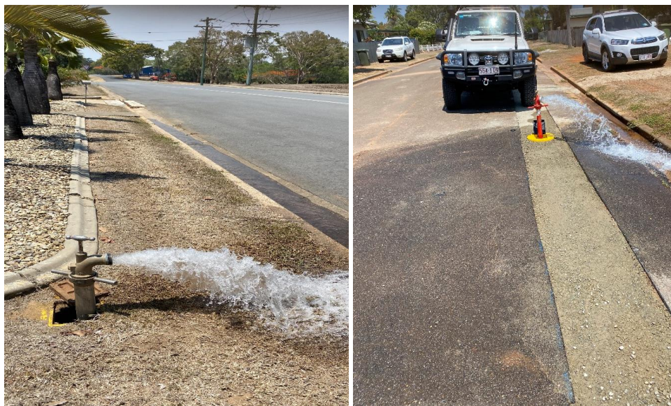
Keeble Street and Adams Street installation of the new 150mm diameter PVC Super-main water main completed
