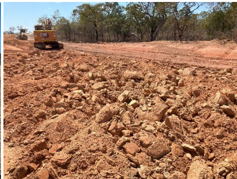
Broken rock prior to table drain clearing
