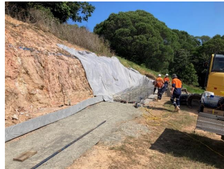
Gabion wall first layer underway
