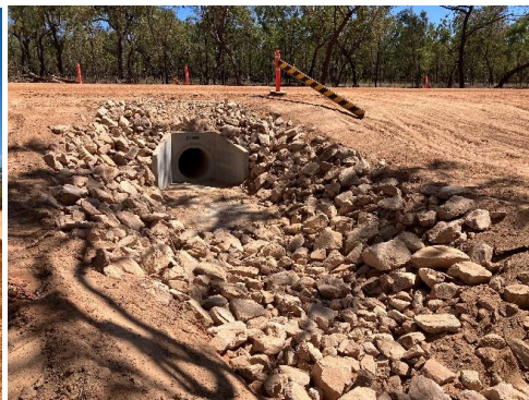
Rock protection to RCP culvert outlet
