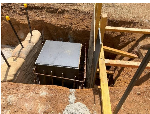
Drop box fabrication
