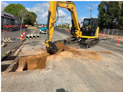
Storm water trenching
