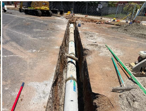
Storm water installation
