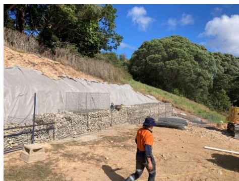
Gabion wall second layer underway
