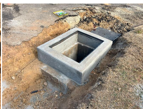
Completed drop box
