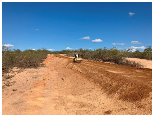
Embankment to subgrade
