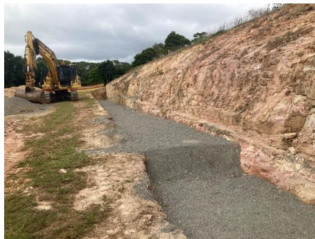
Gabion wall foundation construction
