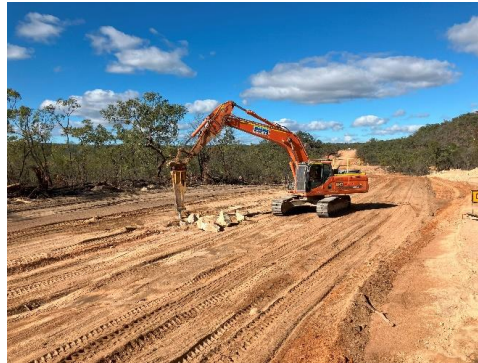
Rock breaker bringing road down to subgrade level
