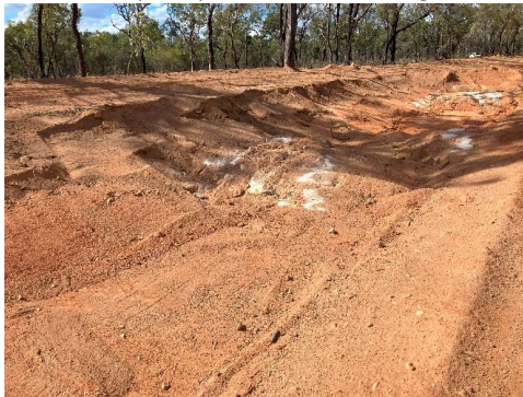
Exposed rock in table drains
