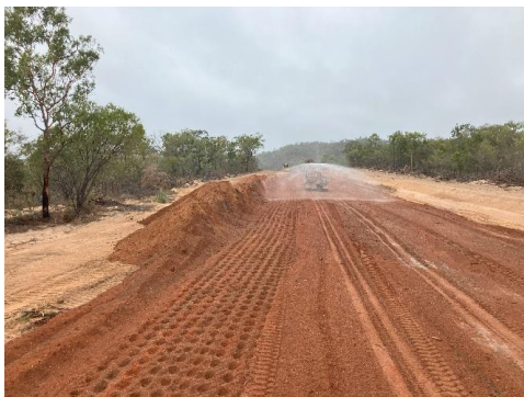
Embankment filling operation
