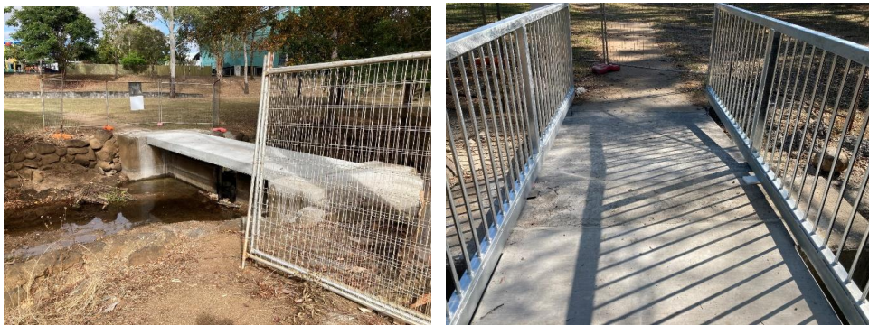
Construction of the new accessible footbridge
