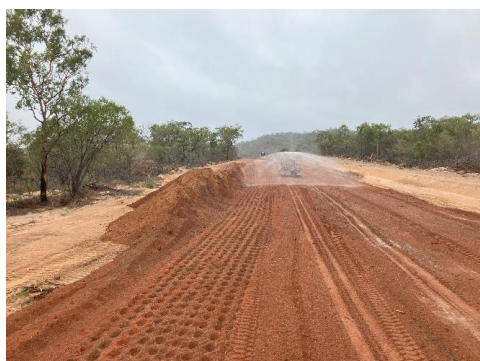
Embankment filling operation
