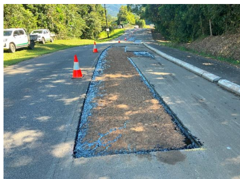
Milled section prepped for asphalt
