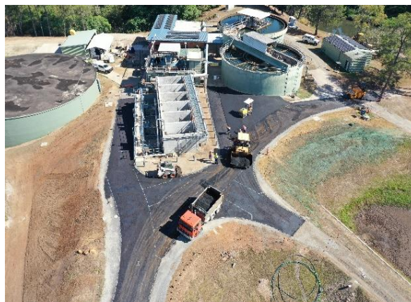
Installation and reinstatement of road pavement
