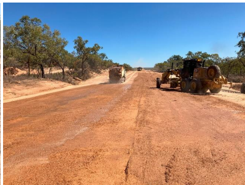
Earthworks to subgrade level
