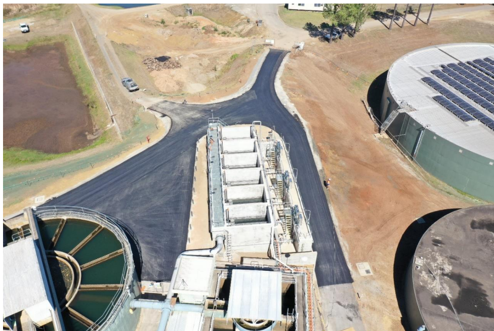
Installation and reinstatement of road pavement
