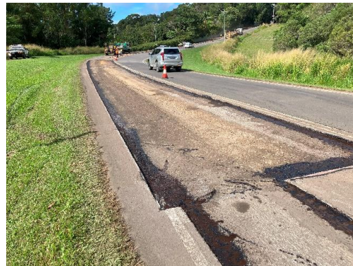
Milled section prepped for asphalt
