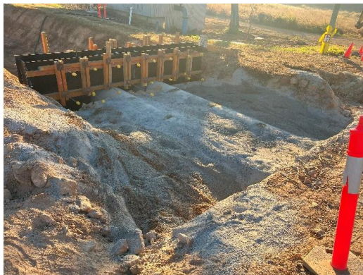
Widening existing channel overflow crossing
