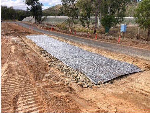
Treating failed subgrade section
