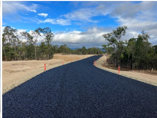
Section 1 seal complete
