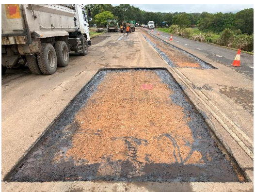
Milled patch prior to asphalt filling
