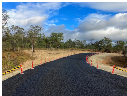
Section 3 seal complete
