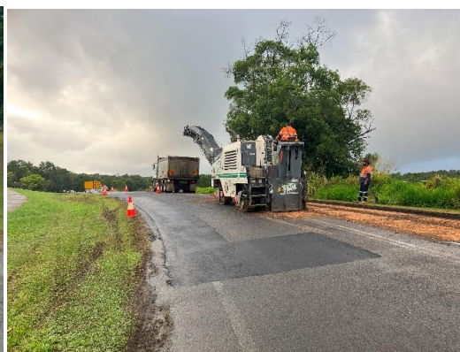
Milling of failed section
