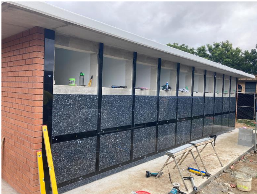
Mareeba Cemetery Mausoleum Wall Construction Nearing Completion
