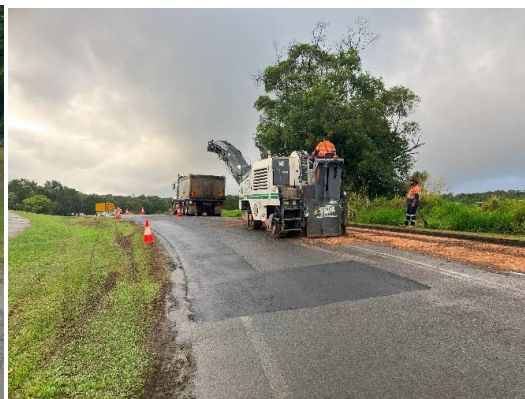
Milling of failed section
