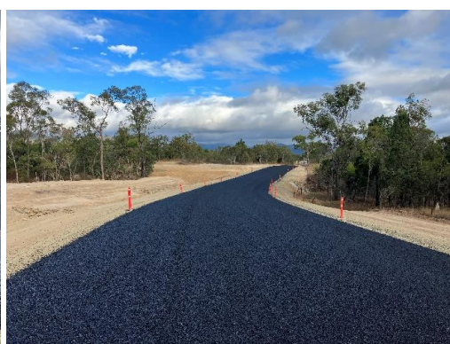
Section 1 seal complete
