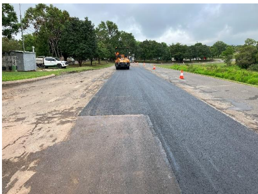
Compaction of asphalt filling
