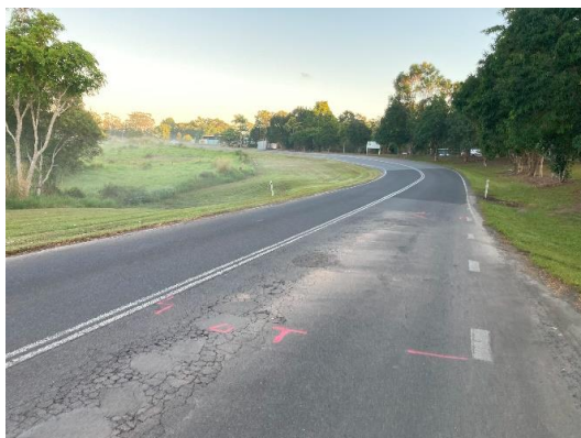
Example of pavement failure on Myola Road
