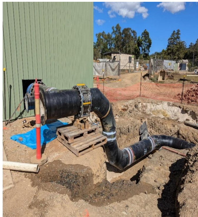
Site construction works and electrical and mechanical fit out underway.
