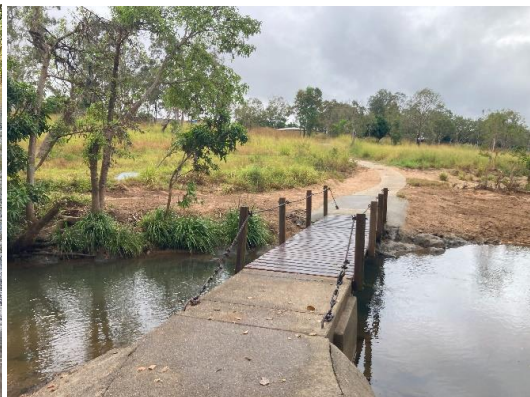
Pedestrian bridge after repair
