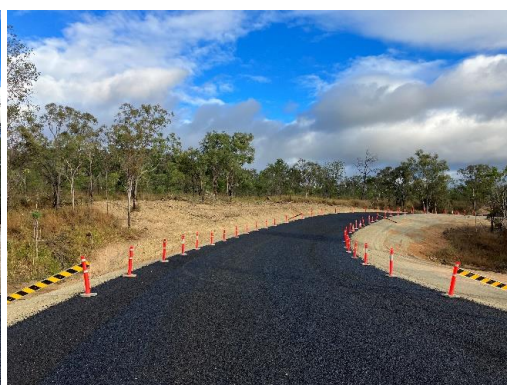
Section 3 seal complete
