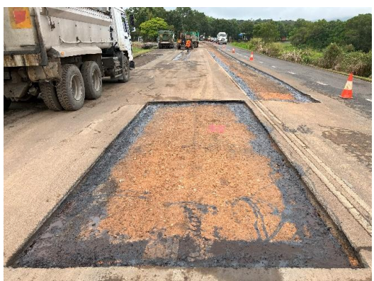
Milled patch prior to asphalt filling
