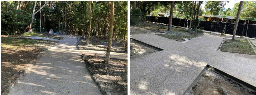
Upgrade footpaths and picnic setting slabs
