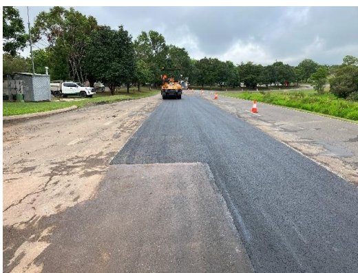
Compaction of asphalt filling
