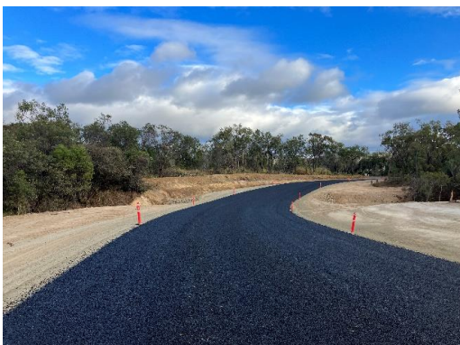
Section 2 seal complete
