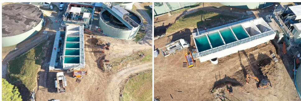
Concrete construction of new filter cell modules and installation of new pipe work and earth works to back fill around the filtration modules.
