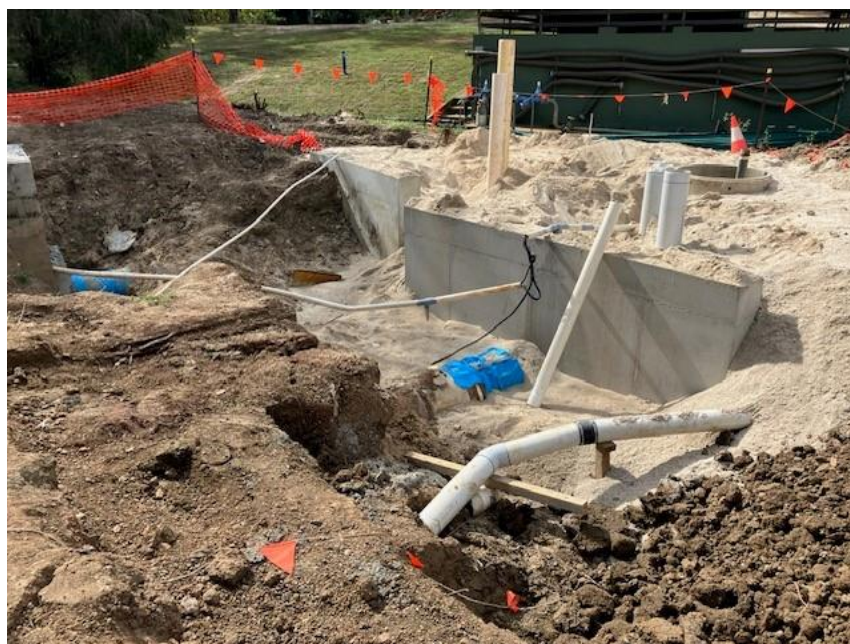
Site construction works and concrete plinth for booster pumps to be mounted onto.
