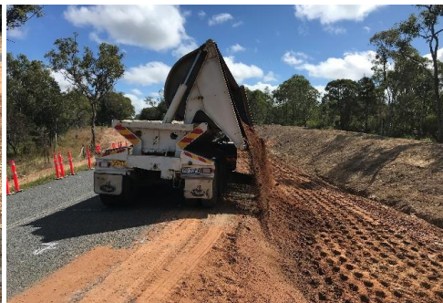
Commencement of earthworks
