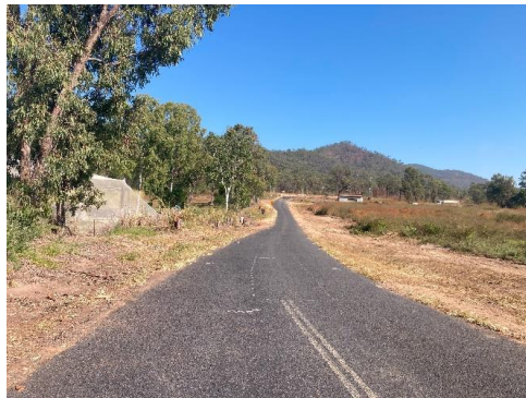
Clearing and grubbing on Springmount Road
