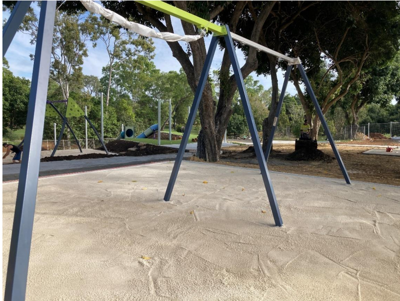
Bicentennial Lakes Mason Street Playground Construction – Swing
