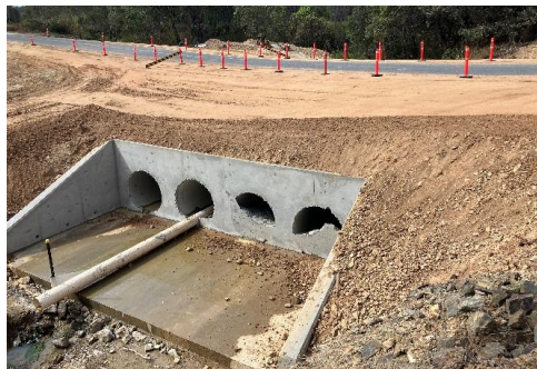
Culvert C1-C2 completed
