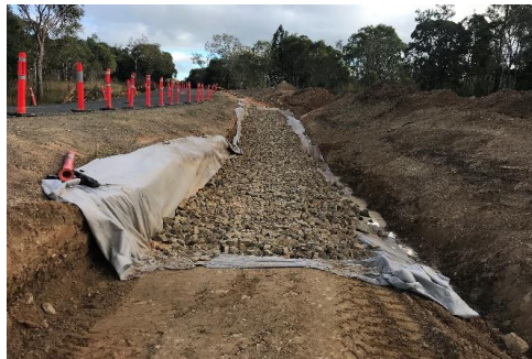
Bidum and rock unsuitable subgrade treatment
