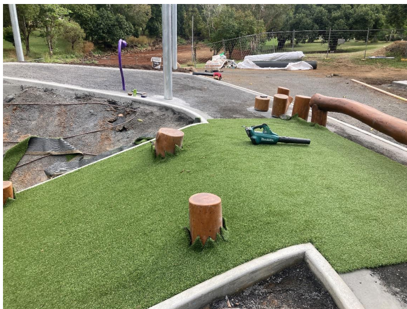
Bicentennial Lakes Mason Street Playground Construction – Hill Slides
