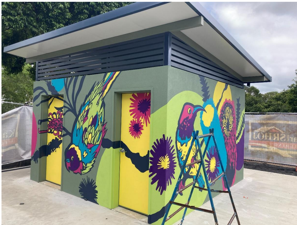
Bicentennial Lakes Southern Section New Public Toilet Construction
