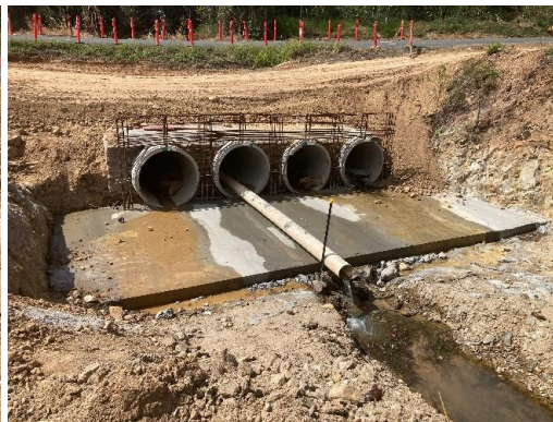
Culvert C1-C2 after apron installation
