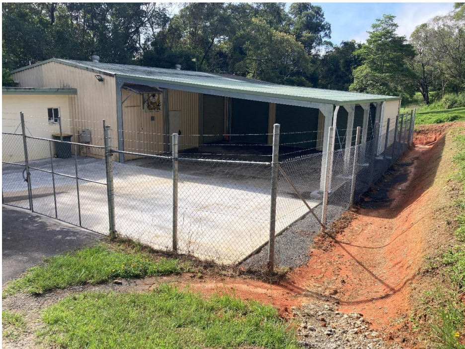
Kuranda SES Facility Skillion Roof, Slab and Drainage improvement Completion
