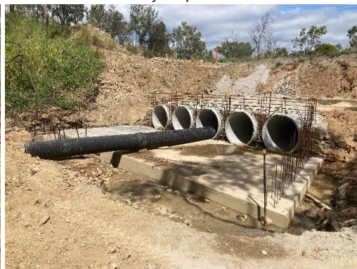
Culvert B after apron installation
