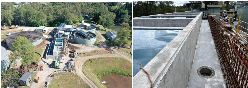
Concrete construction of new filter cell modules and launders
