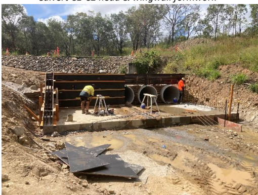
Culvert B head & wingwall formwork
