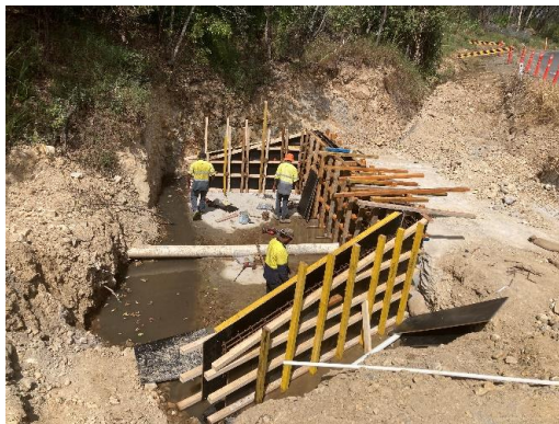
Culvert C1-C2 head & wingwall formwork
