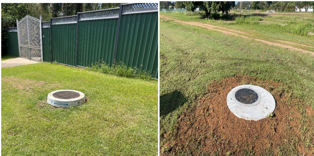
Sewer manhole remediation works
