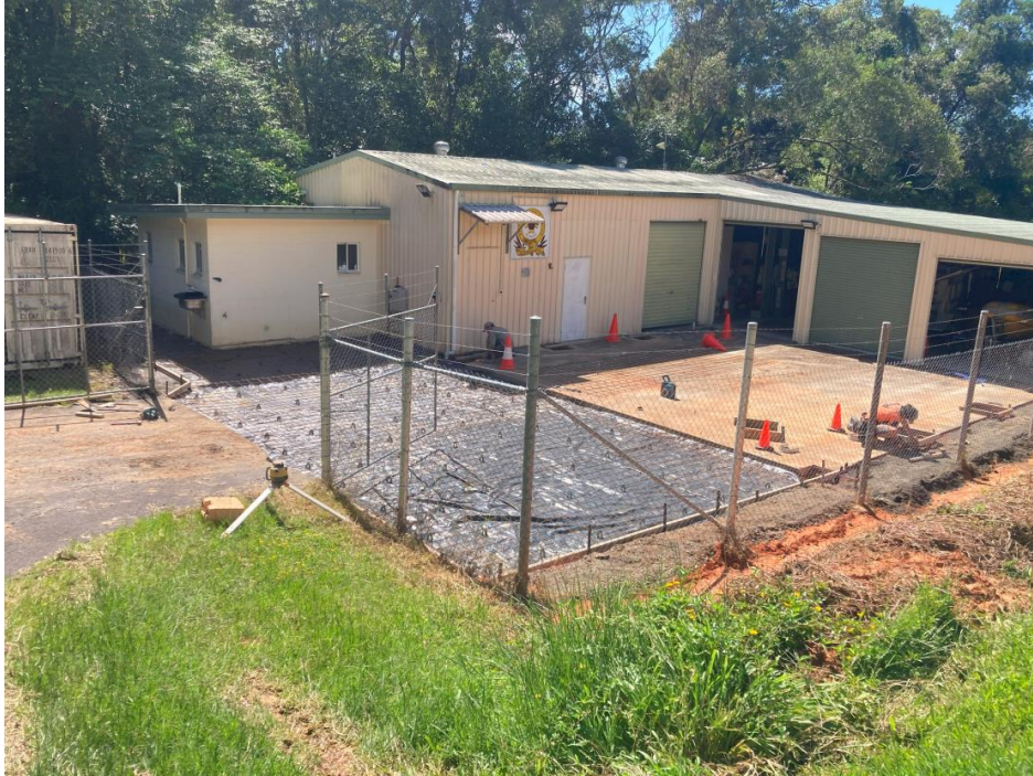
Kuranda SES Facility – Concrete Slab Construction
