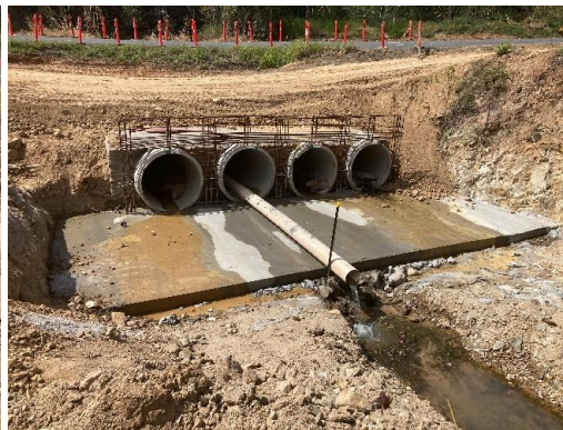
Culvert C1-C2 after apron installation
