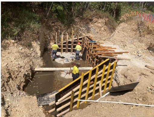
Culvert C1-C2 head & wingwall formwork
