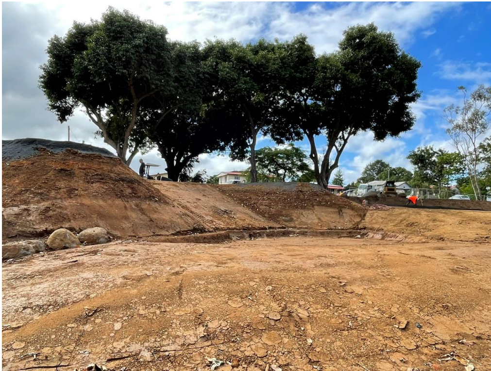
Bicentennial Lakes Playground Construction – Hill Slides
