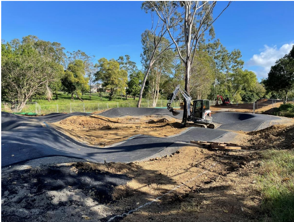
Bicentennial Lakes Pump Track Construction
