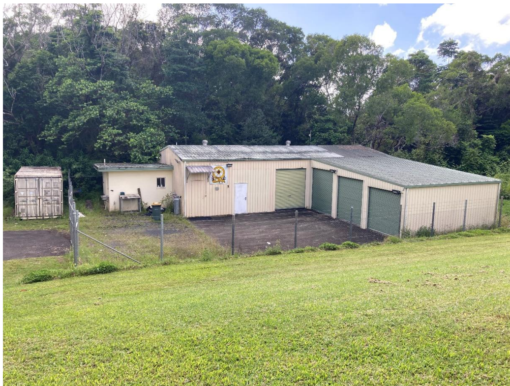
Kuranda SES Facility Prior to Upgrade Works
