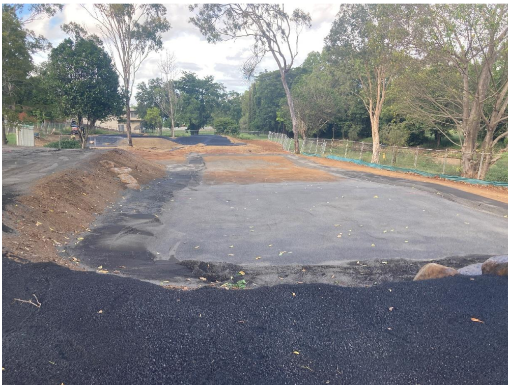
Bicentennial Lakes Playground Construction – Flying Fox
