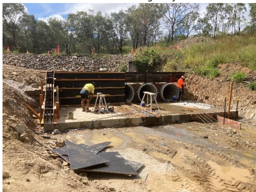
Culvert B head & wingwall formwork
