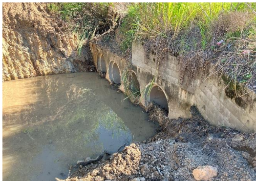
Culvert C1-C2 prior to extension
