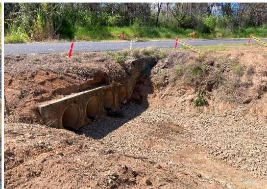
Culvert C1-C2 after earthworks
