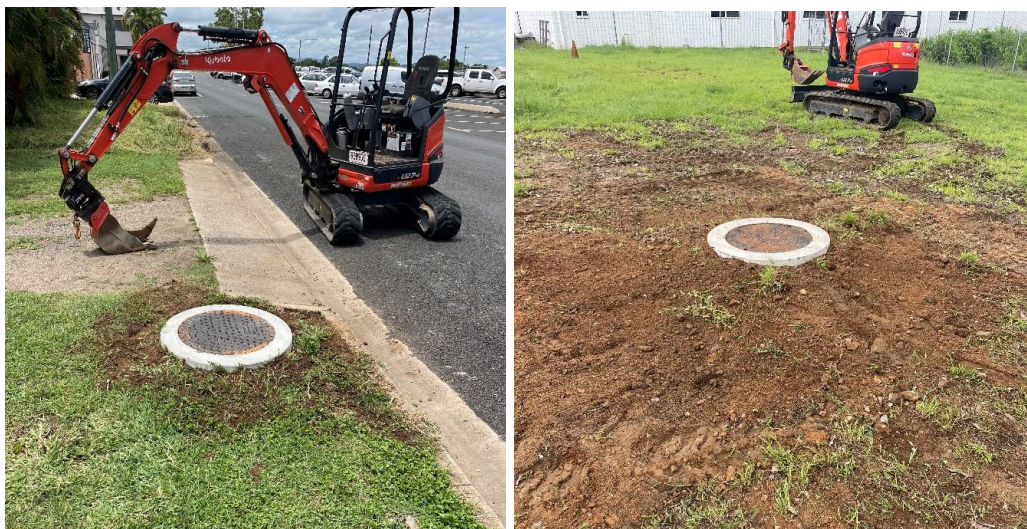
Sewer manhole remediation works
