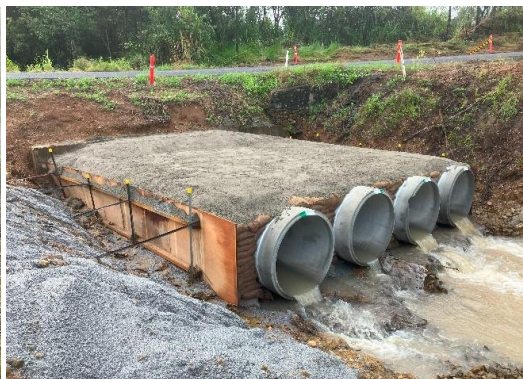
Culvert C1-C2 functioning
