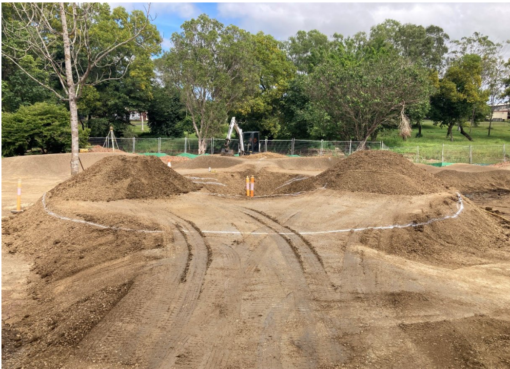
Bicentennial Lakes Pump Track Construction
