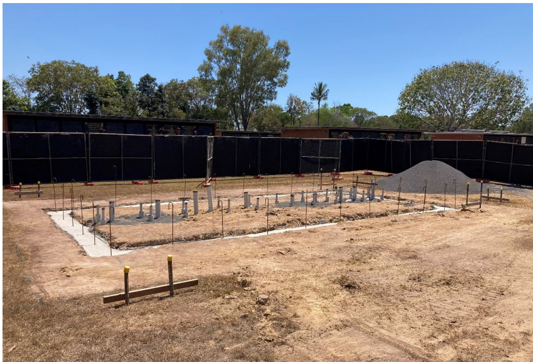
Mausoleum Wall Footings Construction
