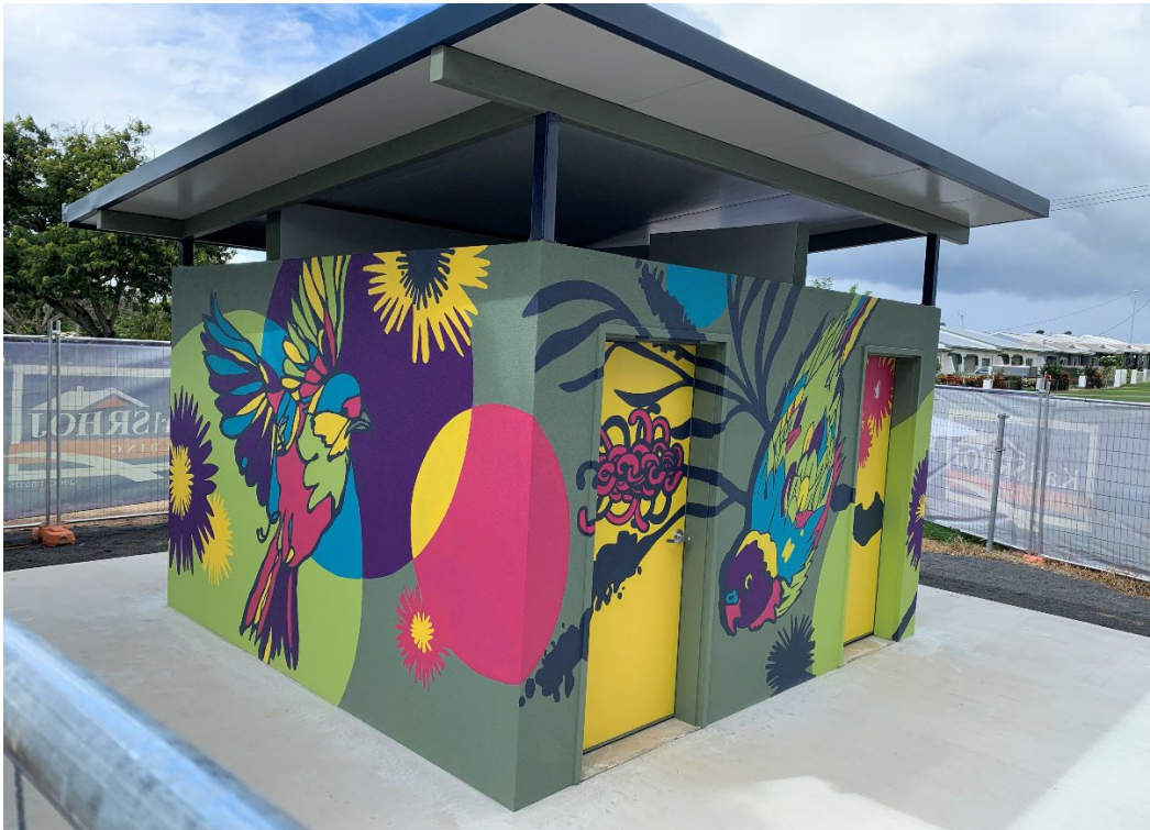
Bicentennial Lakes Southern Section New Public Toilet Construction
