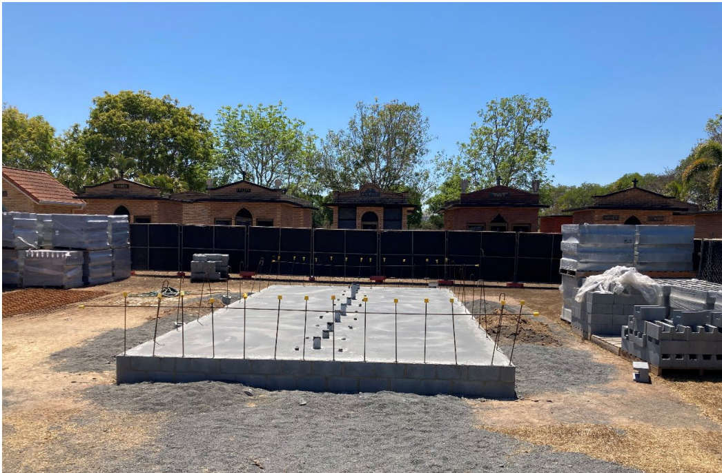
Mausoleum Wall Concrete Pad Construction
