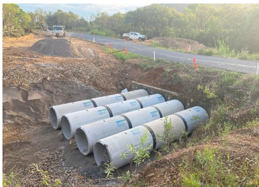
Culvert C1-C2 prior to backfilling with stabilised sand
