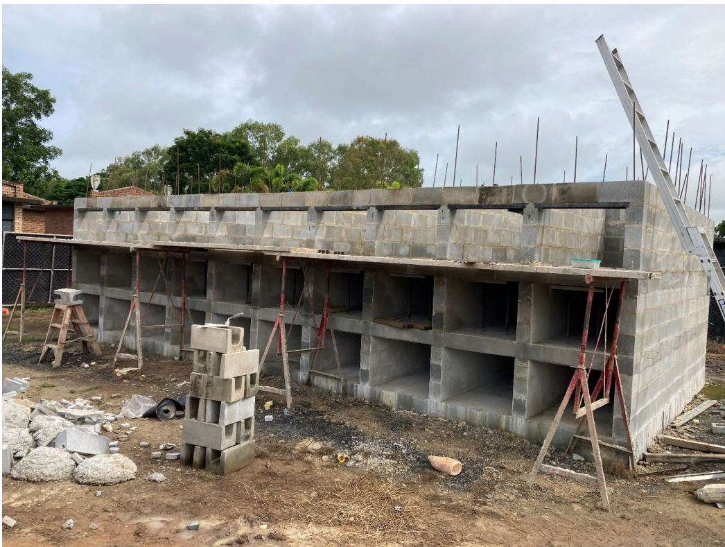
Mausoleum Wall Construction
