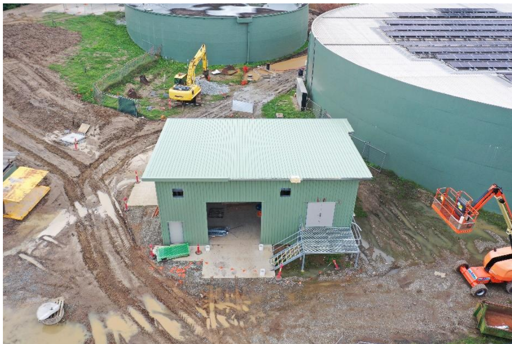
Site building construction works and fire suppression equipment and booster pumps.
