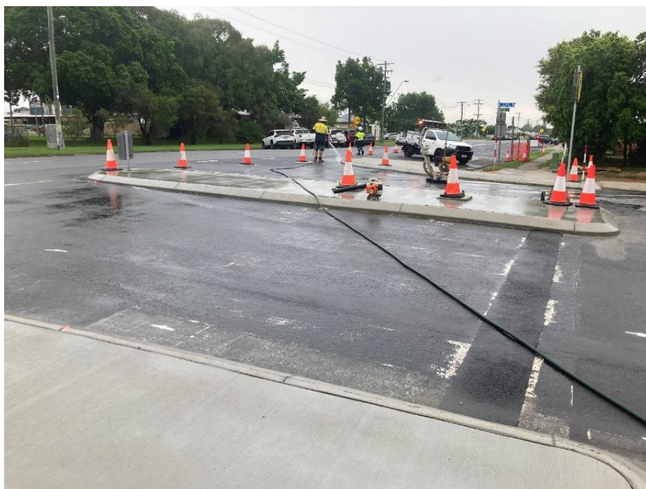
Concrete island infill
