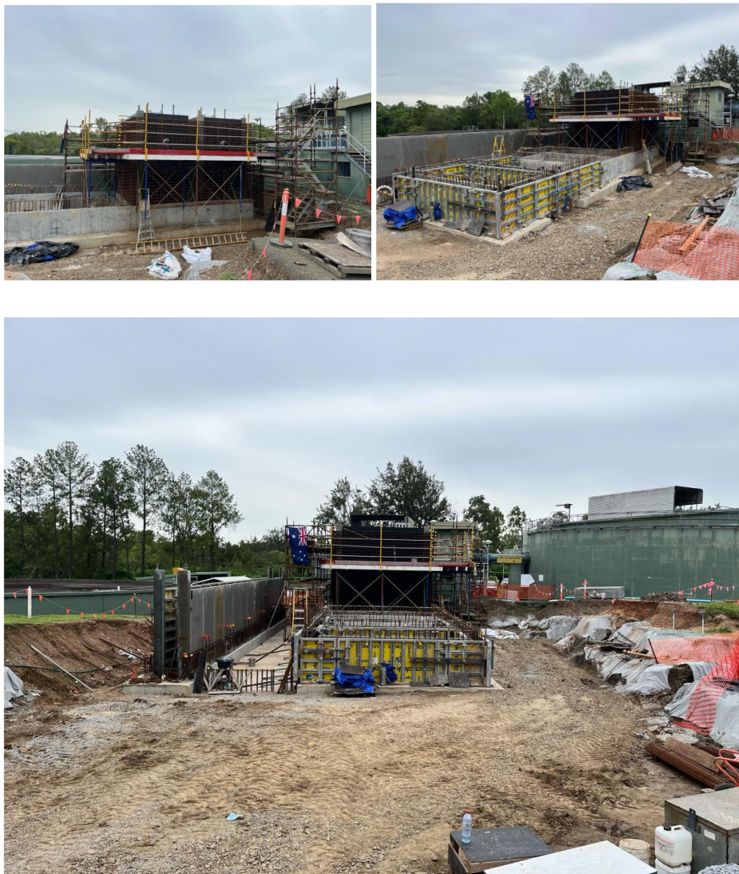
Concrete construction of new filter cell modules.
