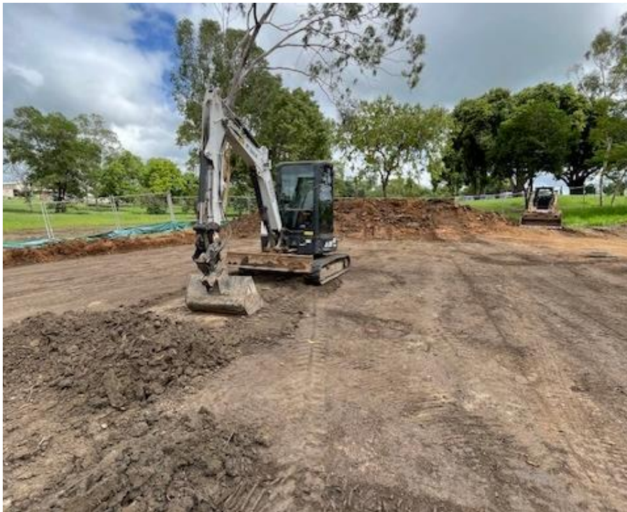
Bicentennial Lakes Pump Track Site Preparation
