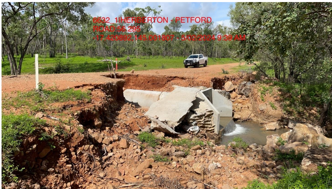
Culvert washout on Herberton-Petford Road
