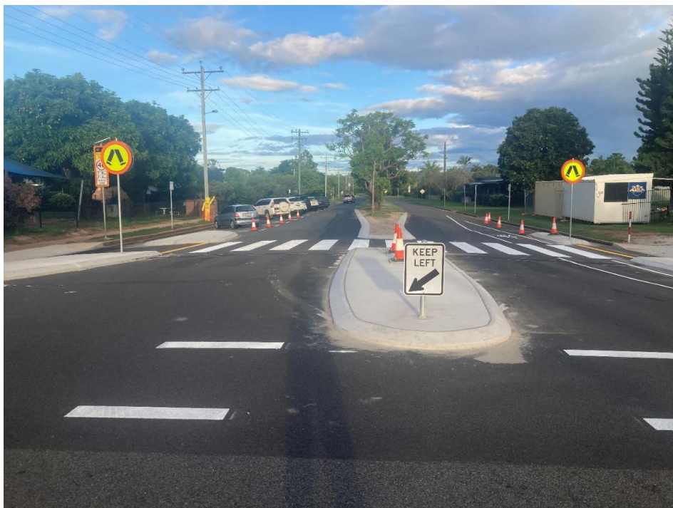
After - Completion of Pavement Marking
