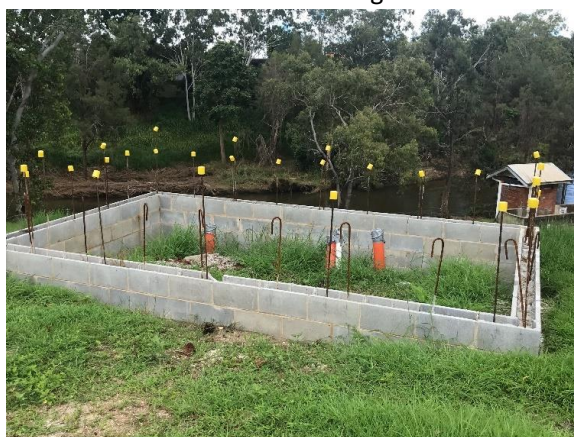
Electrical cabling conduits installed
