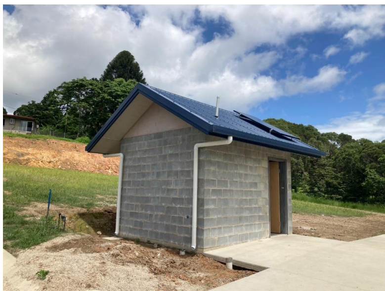
Kuranda Heights Cemetery – New footpath complete and toilet construction commenced.
