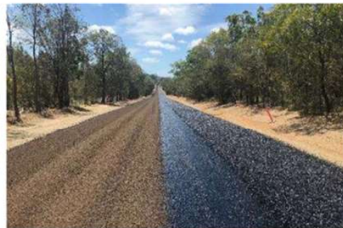
Bitumen sealing (2 nd coat)
