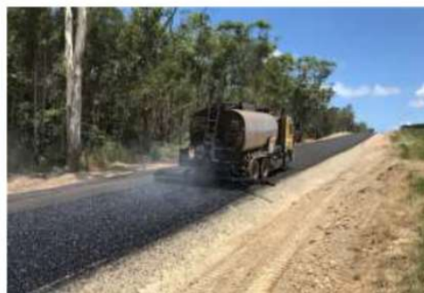
Bitumen Sealing (2 nd Coat)
