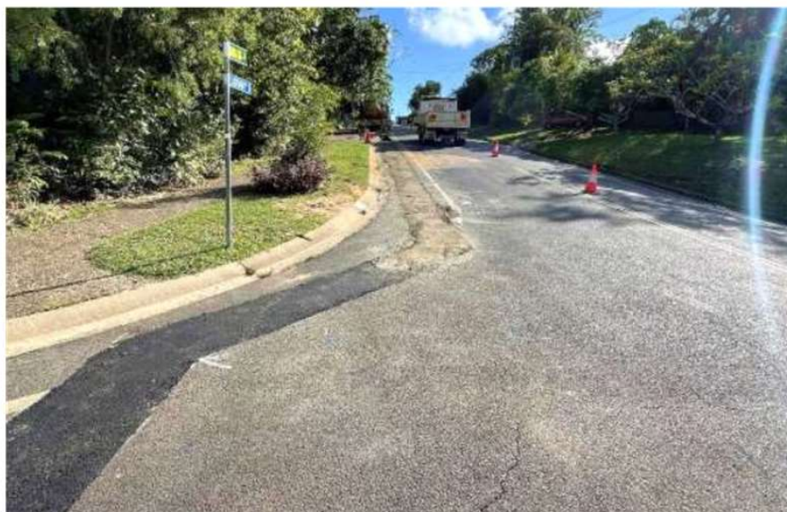
Reinstatement of road surfacing following water main installation
