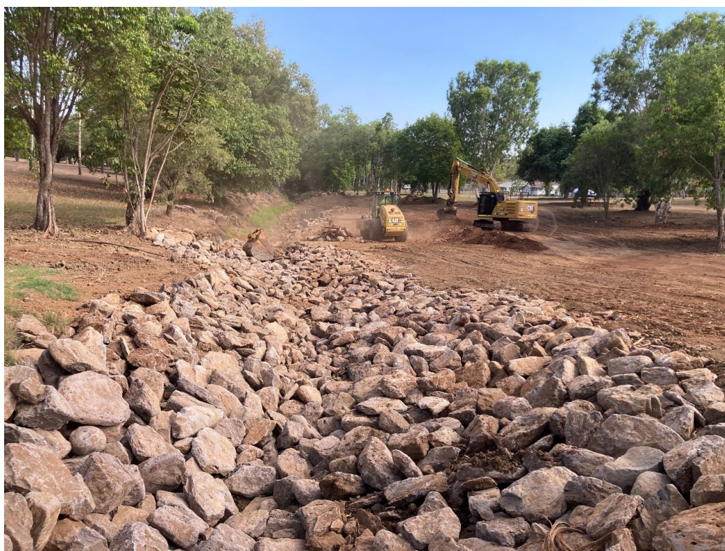
Bicentennial Lakes Southern Section Reconfiguration Rock Lining Installation
