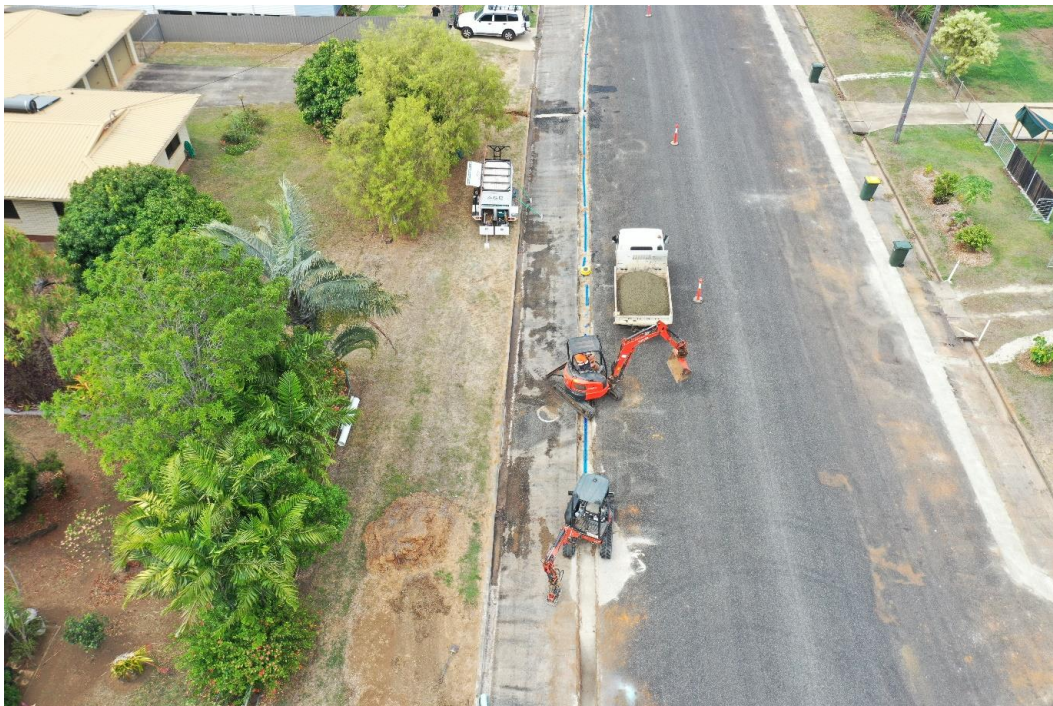
Mason Street installation of the new 150mm diameter PVC Supermain water main
