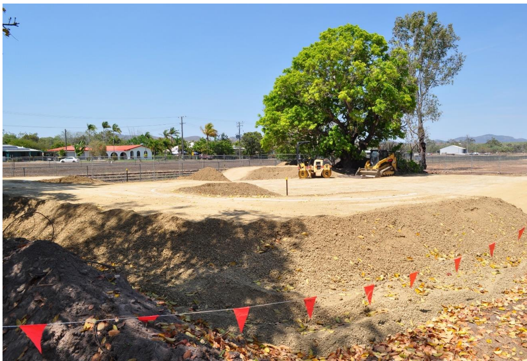
Dimbulah Pump Track Shaping Earthworks
