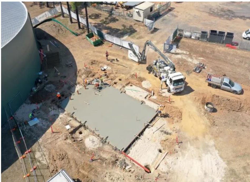
Concrete pour for main slab of booster pump station building
