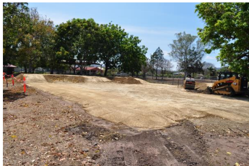
Dimbulah Pump Track Shaping Earthworks
