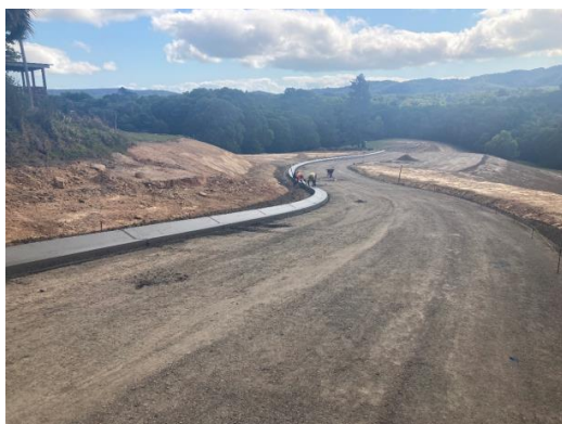
New Kuranda Cemetery – Kerb Installation
