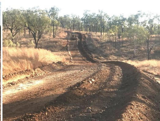
Laying out re-sheet material
