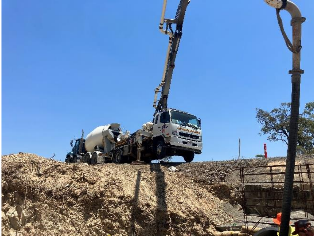
Pumping concrete for culvert apron
