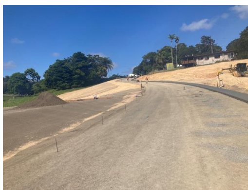
New Kuranda Cemetery – Kerb Installation
