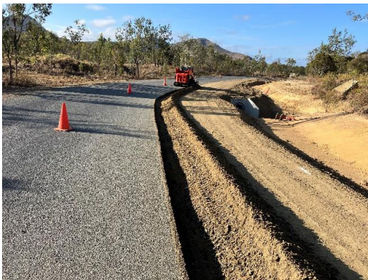
Milling out existing pavement
