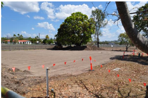
Dimbulah Pump Track Foundation Earthworks
