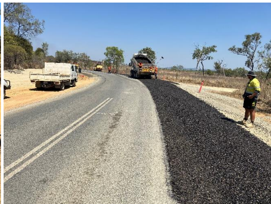
Sealing of pavement widening
