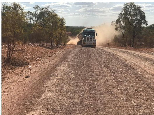
Side tipping truck delivering material to the road
