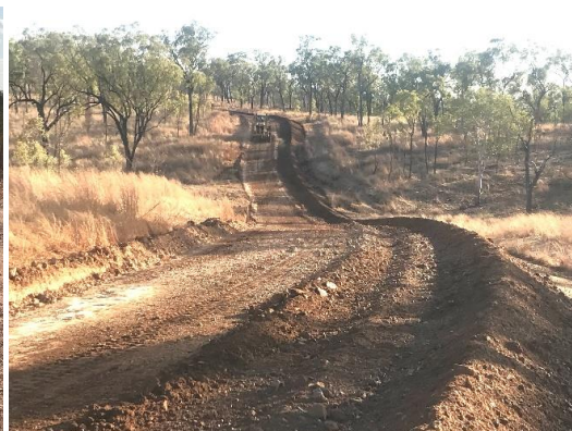
Laying out re-sheet material
