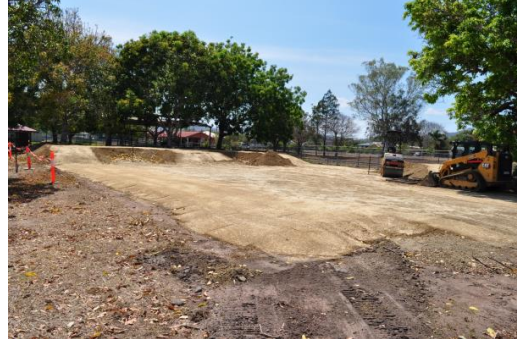
Dimbulah Pump Track Shaping Earthworks
