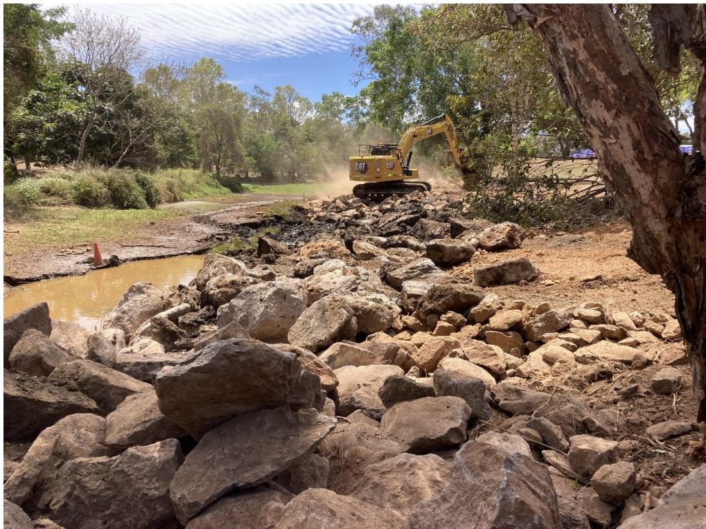
Bicentennial Lakes Southern Section Reconfiguration Rock Lining Installation
