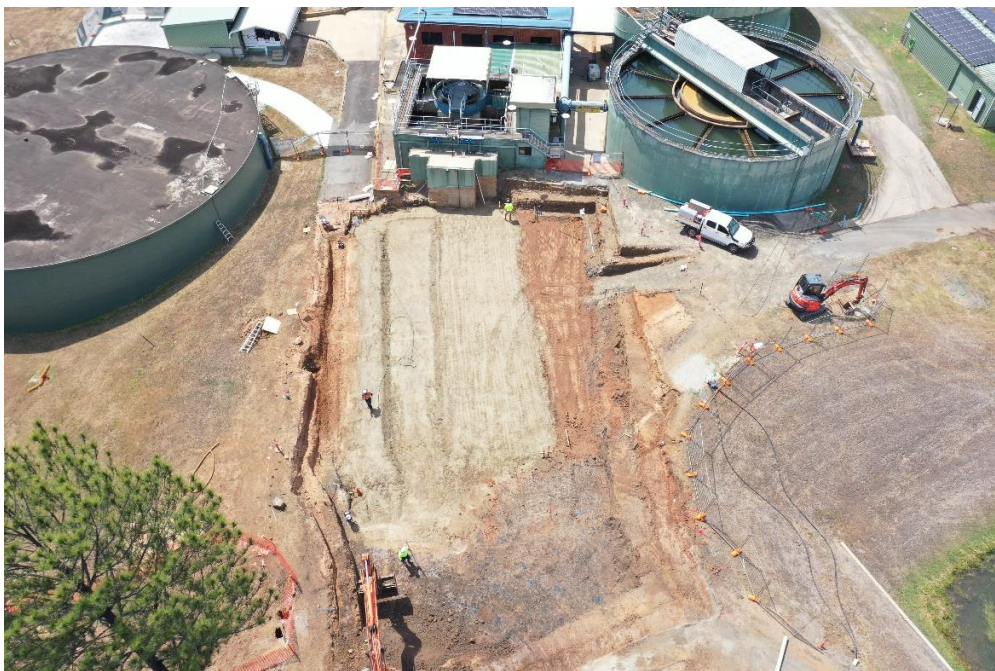
Civil earthworks for new filtration system
