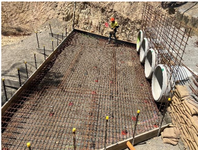
Culvert apron prior to pouring
