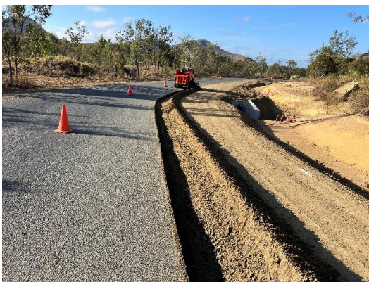
Milling out existing pavement
