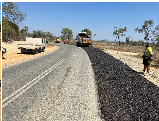
Sealing of pavement widening
