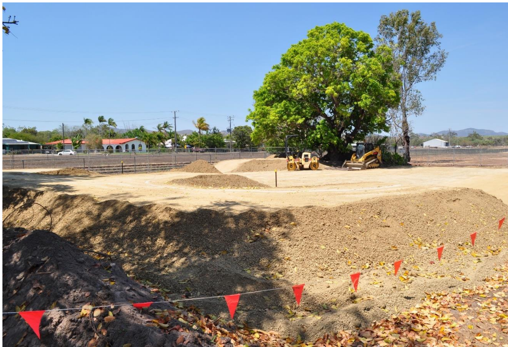
Dimbulah Pump Track Shaping Earthworks
