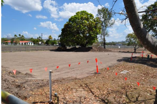
Dimbulah Pump Track Foundation Earthworks
