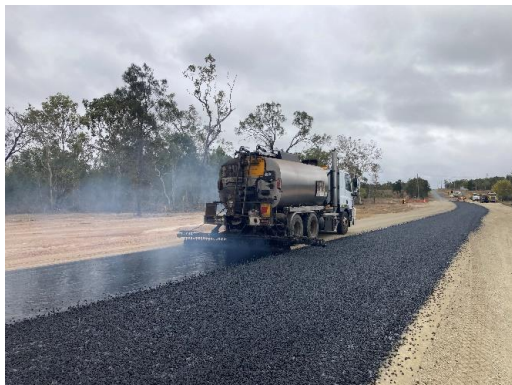
Bitumen seal – first coat (16mm)
