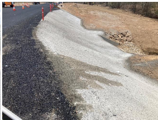
Completed concrete batter protection
