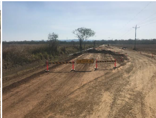
Detour in place
