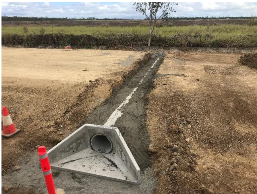
One of four additional culverts
