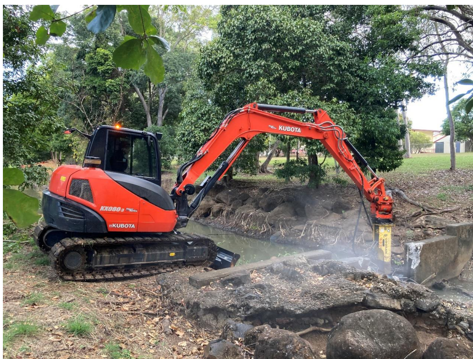
Bicentennial Lakes Southern Section Weir Removal
