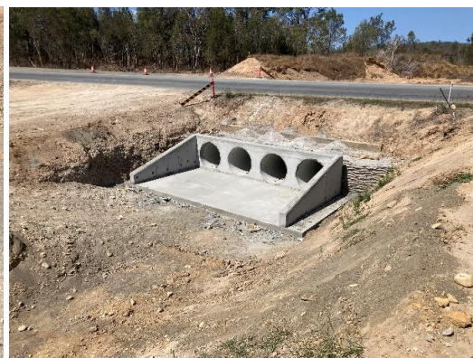
Completed culvert and apron
