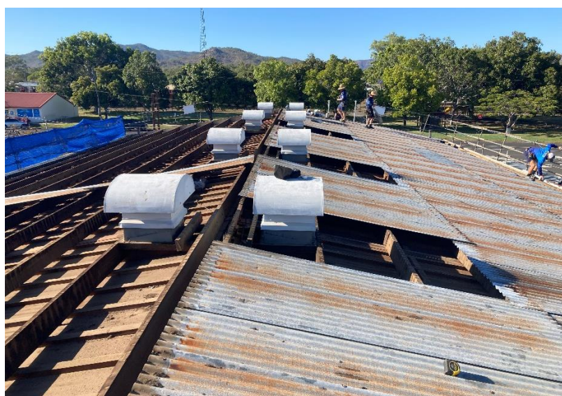
Dimbulah Memorial Hall Roof Replacement and Insulation Upgrade – Project Commencement
