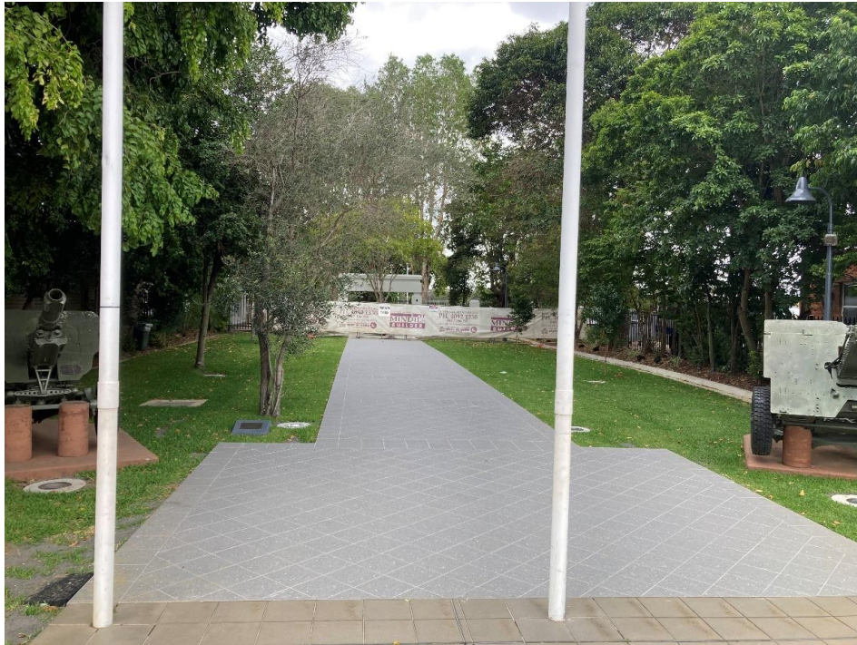
Anzac Park Footpath Replacement –new tiled footpath construction
