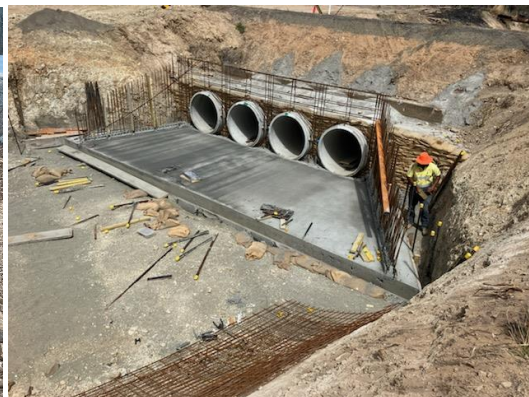
Culvert headwall and apron construction
