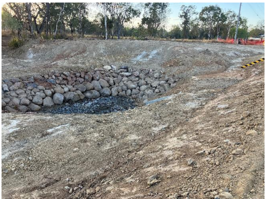
Rock protection works
