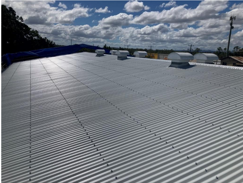
Dimbulah Memorial Hall Roof Replacement and Insulation Upgrade – Project Completion
