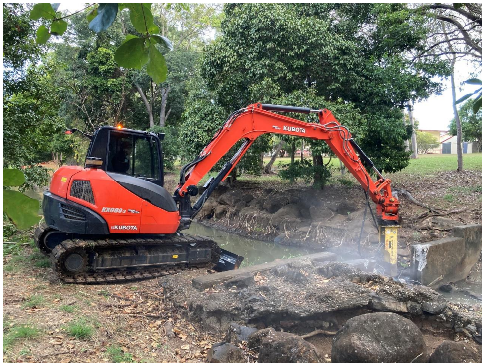
Bicentennial Lakes Southern Section Weir Removal
