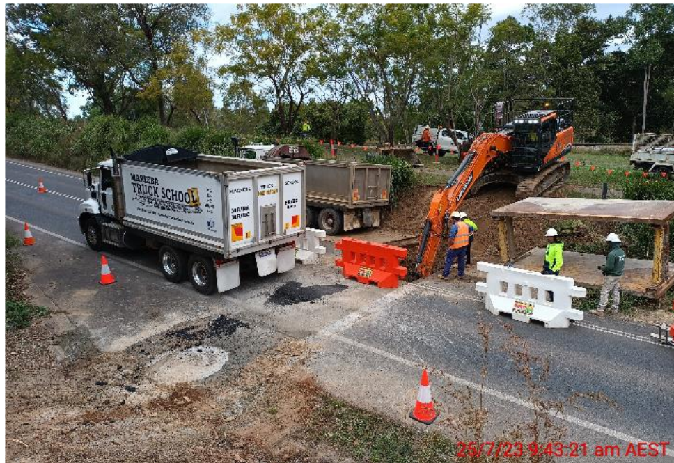
Trenching through Byrnes Street (TMR Corridor) under single lane closure
