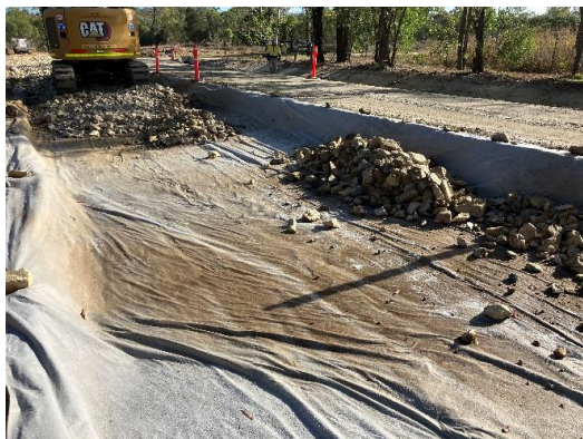
Unsuitable material replacement
