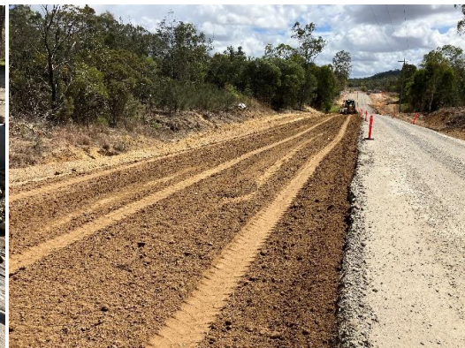
Subbase layer installation
