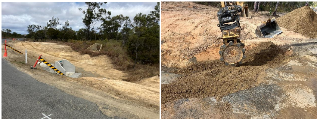
Installed pre-fabricated headwall
