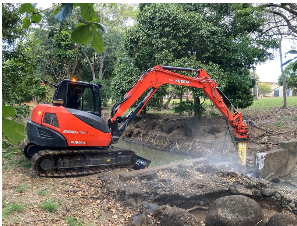
Bicentennial Lakes Southern Section Weir Removal
