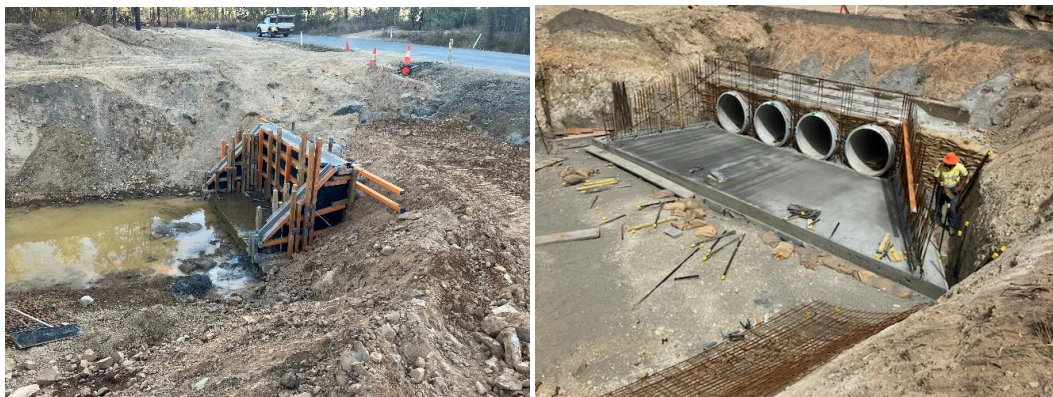
Culvert headwall and apron construction
