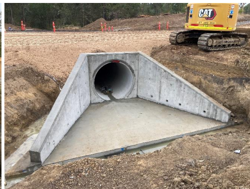
1800Ø RCP headwall complete
