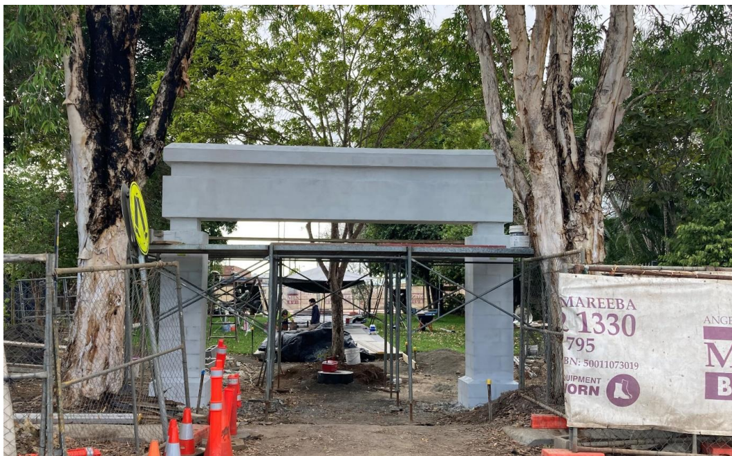
Anzac Park Mareeba Construction Works – Railway Avenue Entrance
