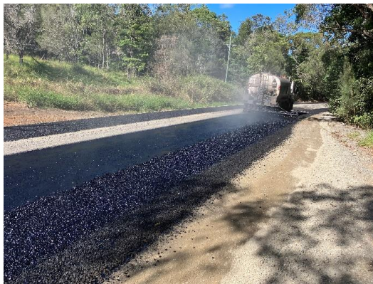
Second coat 10mm seal
