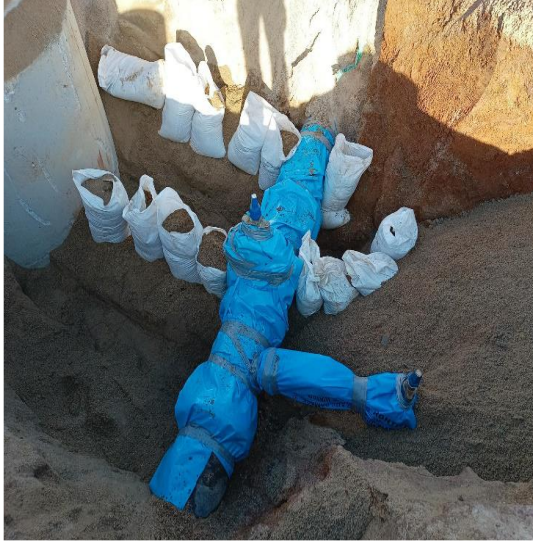
DN300 valve assembly prepped for thrust block concrete pour, and water main marker tape above reinstated DN100 DICL pipe
