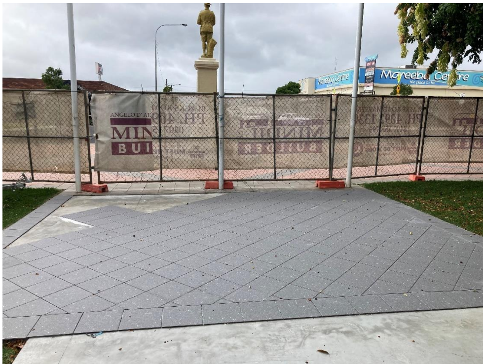
Anzac Park Mareeba Construction Works – Byrnes Street Entrance
