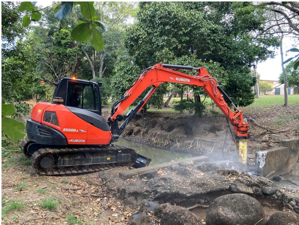
Bicentennial Lakes Southern Section Weir Removal
