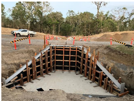
1800Ø RCP headwall after pouring
