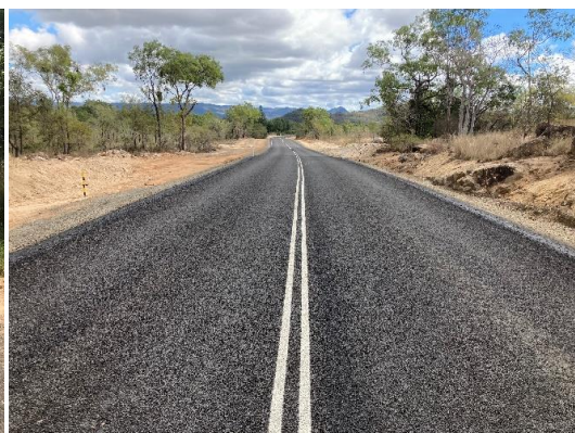
Wolfram Road after
