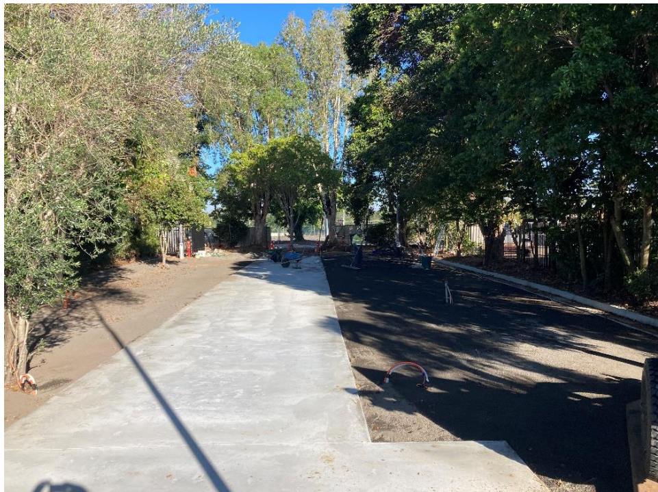
Anzac Park Mareeba Construction Works
