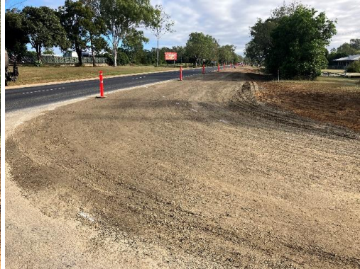
Replaced shoulder material
