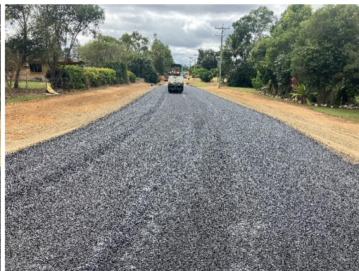
10mm aggregate bitumen seal over full width
