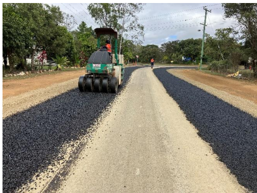
16mm aggregate bitumen seal
