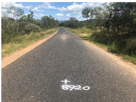
Wolfram Road before
