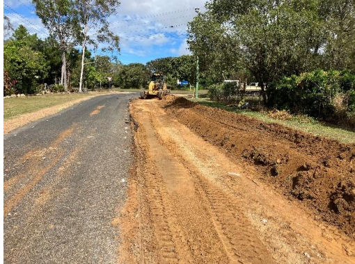
Removing existing shoulder gravel
