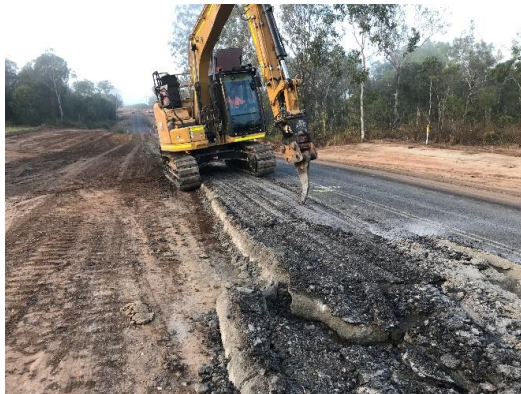
Excavate to new subgrade design
