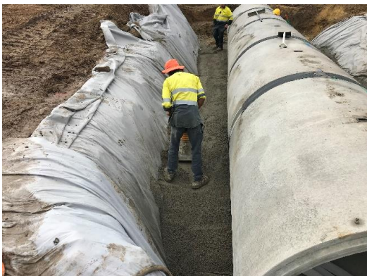
Culvert haunch zone treatment
