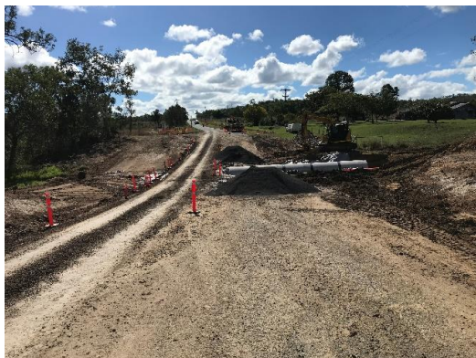
Culvert replacement
