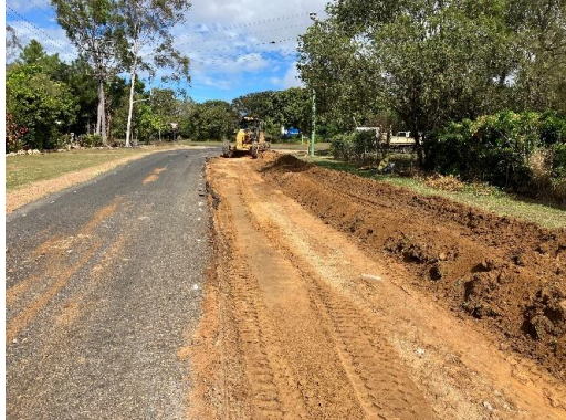
Removing existing shoulder gravel
