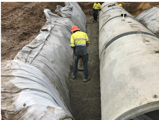
Culvert haunch zone treatment
