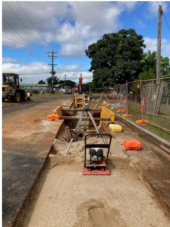
Strattmann Street installation of the new 450mm diameter gravity sewer main
