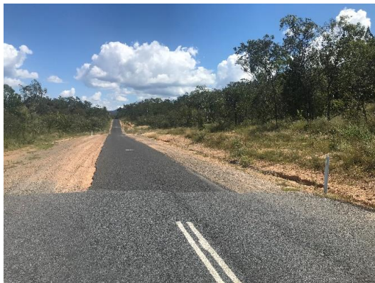
Wolfram Road before
