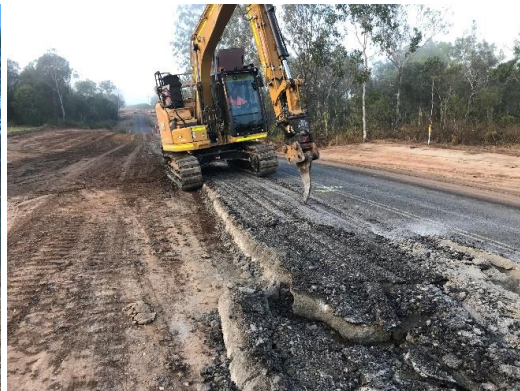
Excavate to new subgrade design
