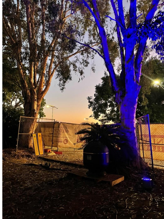
Anzac Park Mareeba Tree Coloured Lighting Test
