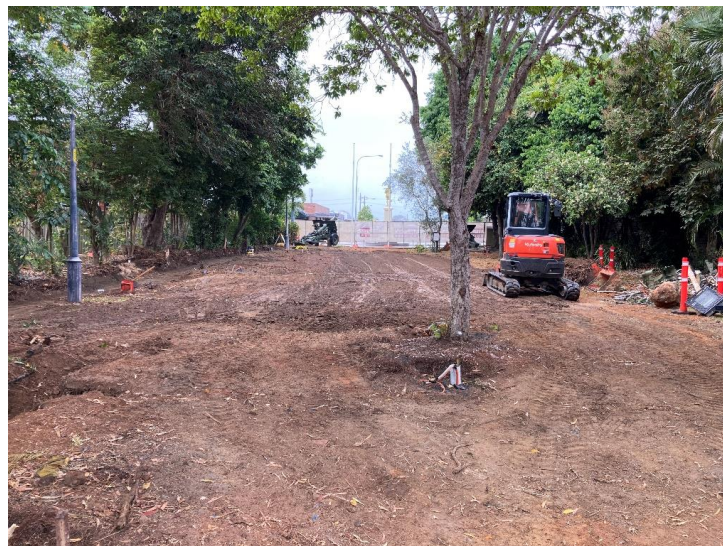
Anzac Park Mareeba Construction Works
