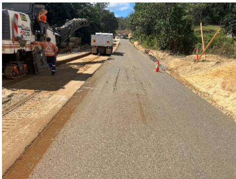
Pavement profiling and filling
