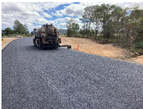
Second coat bitumen sealing
