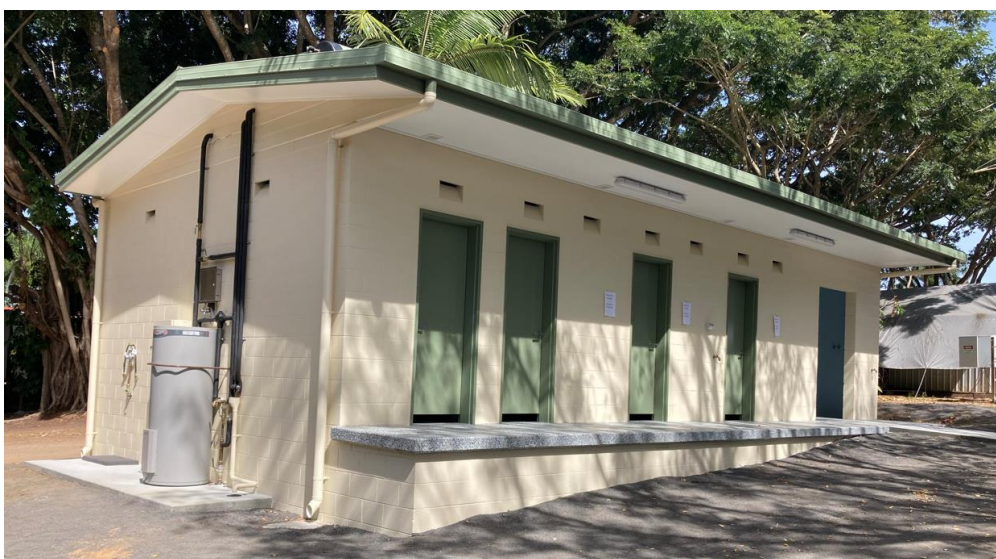
Riverside Caravan Park Amenities block western elevation
