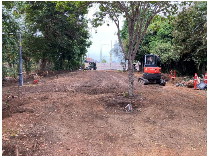
Anzac Park Mareeba Construction Works
