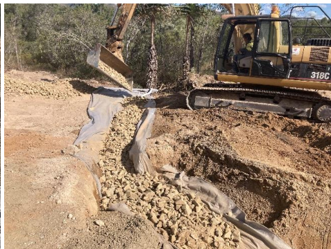
Rock wick drain installation
