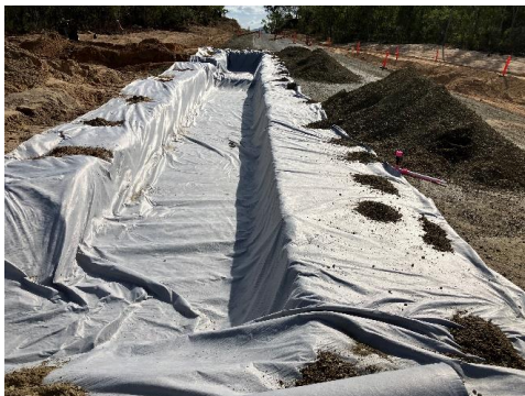
Unsuitable subgrade replacement
