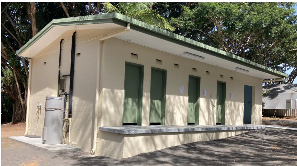
Riverside Caravan Park Amenities block western elevation
