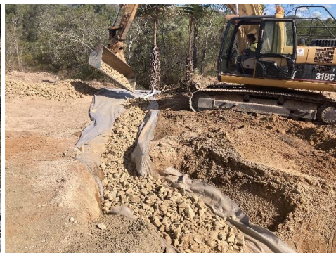
Rock wick drain installation
