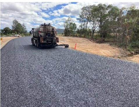
Second coat bitumen sealing
