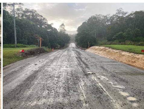
Wet weather is hampering progress
