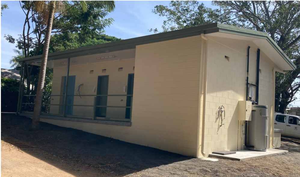
Riverside Caravan Park Amenities block eastern elevation
