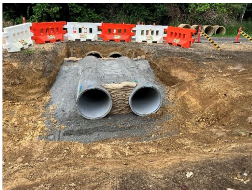
Replacement 1050Ø pipework (Ch 9479)
