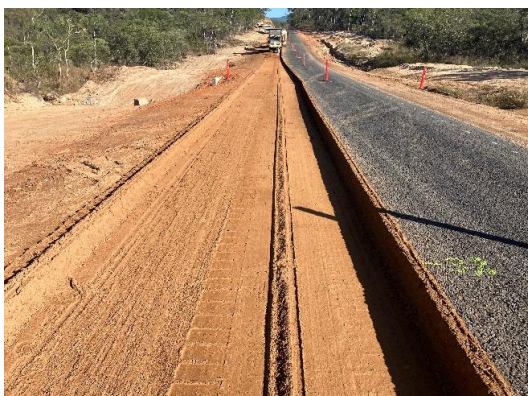
Profiling existing gravel shoulders
