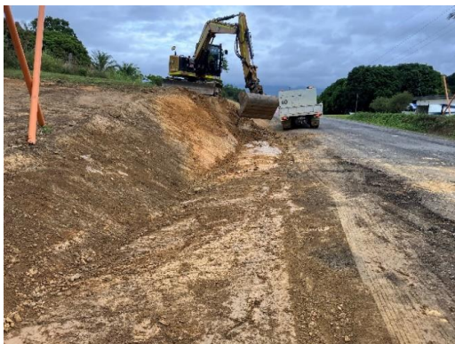
Completing clearing and grubbing
